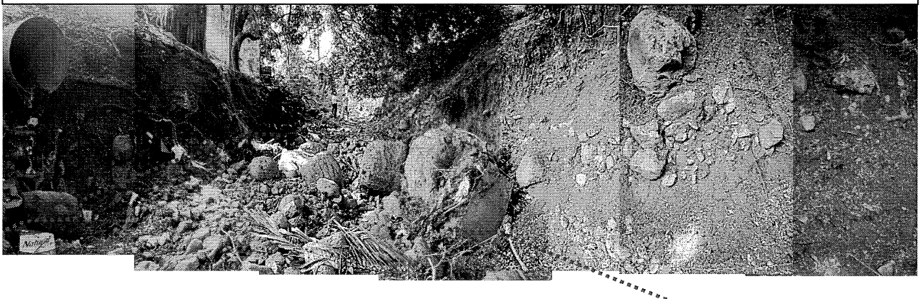
Figure 3 Aiea Stream Location 1. Top: Up-stream view showing right bank (left side of photo) proposed for shotcrete stabilization. Bottom: Downstream view same location. Note line of river rock mid-face on right bank and absence of roots on face of right bank.
