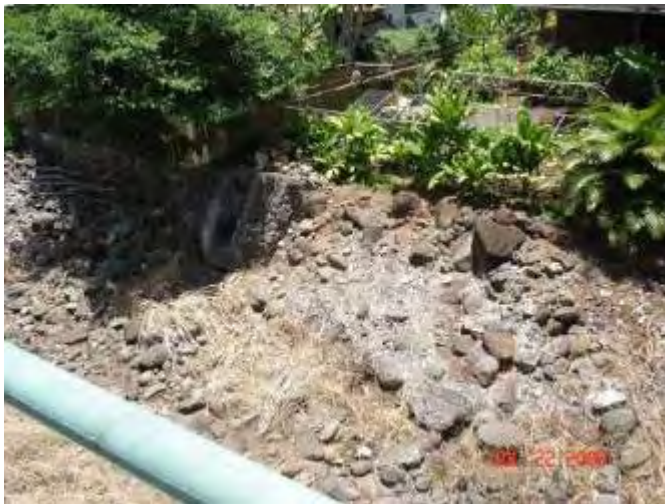
Figure 10. Rubble Wall at Station 300+68 to 300+16.
