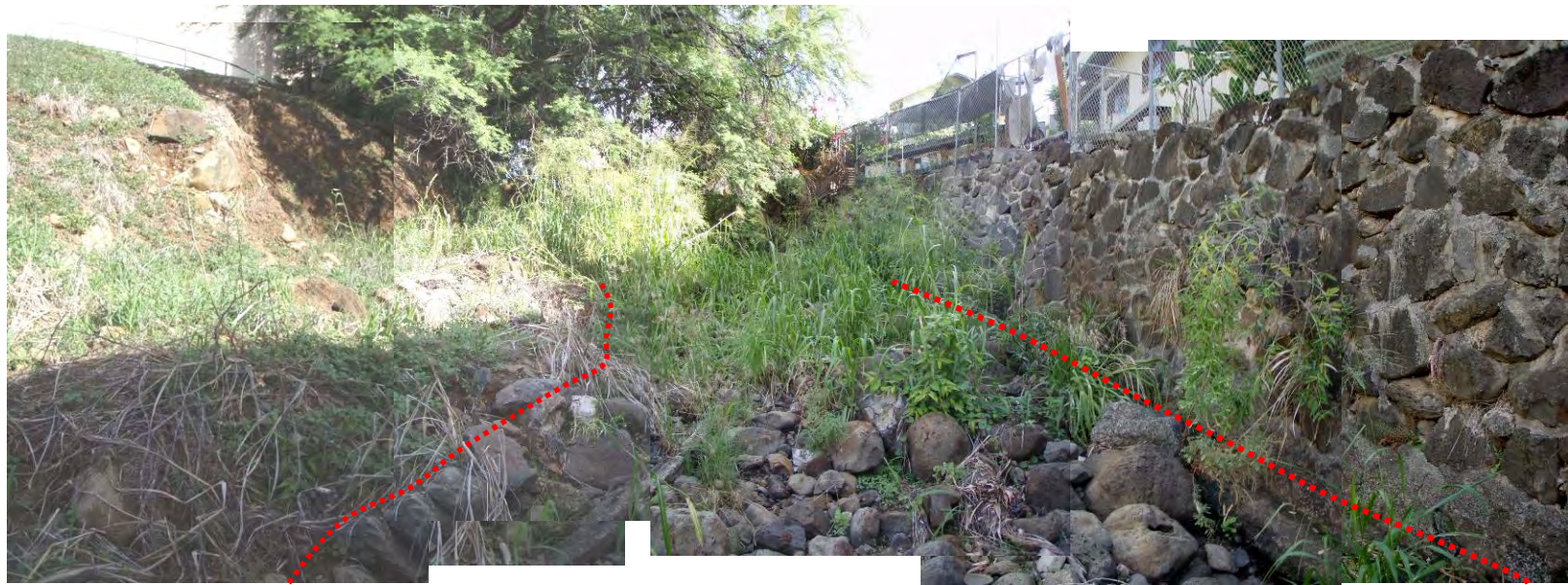
Figure 5 Stream bed at Station 303+40 about 100 feet below lower end of project site. Top: Upstream view. Large tree in background left marks lower end of proposed shotcrete wall on right bank. Note undermining of rock wall on left bank (right side upper photo). Bottom: Downstream view from same location showing grass slope on right bank and vertical concrete reinforced rock wall on left bank. Dashed red line represents approximate OHWM.
