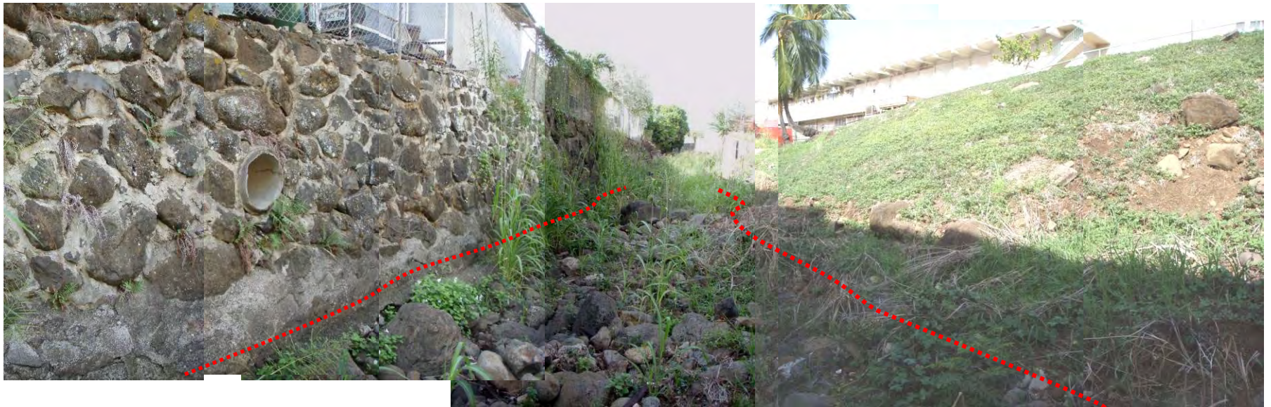
Figure 5 Stream bed at Station 303+40 about 100 feet below lower end of project site. Top: Upstream view. Large tree in background left marks lower end of proposed shotcrete wall on right bank. Note undermining of rock wall on left bank (right side upper photo). Bottom: Downstream view from same location showing grass slope on right bank and vertical concrete reinforced rock wall on left bank. Dashed red line represents approximate OHWM.
