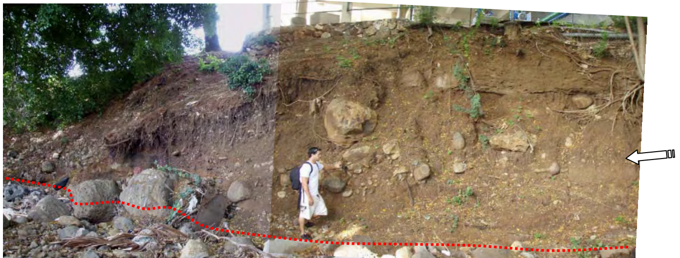
Figure 3 Right Bank near center of proposed project. Note line of rounded "river rock" embedded in bank from arrow to hand indicating possible historical elevation of a portion of the stream bed. Unlayered dirt and angular rocks above this elevation are indicative of fill. OHWM shown as dotted red line.
