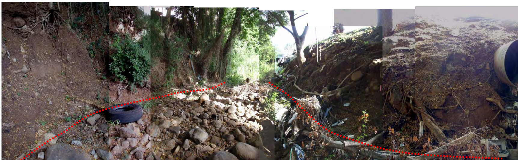
Figure 4 Aiea Stream Location 1. Top: Up-stream view showing right bank (left side of photo) proposed for shot-crete stabilization.
