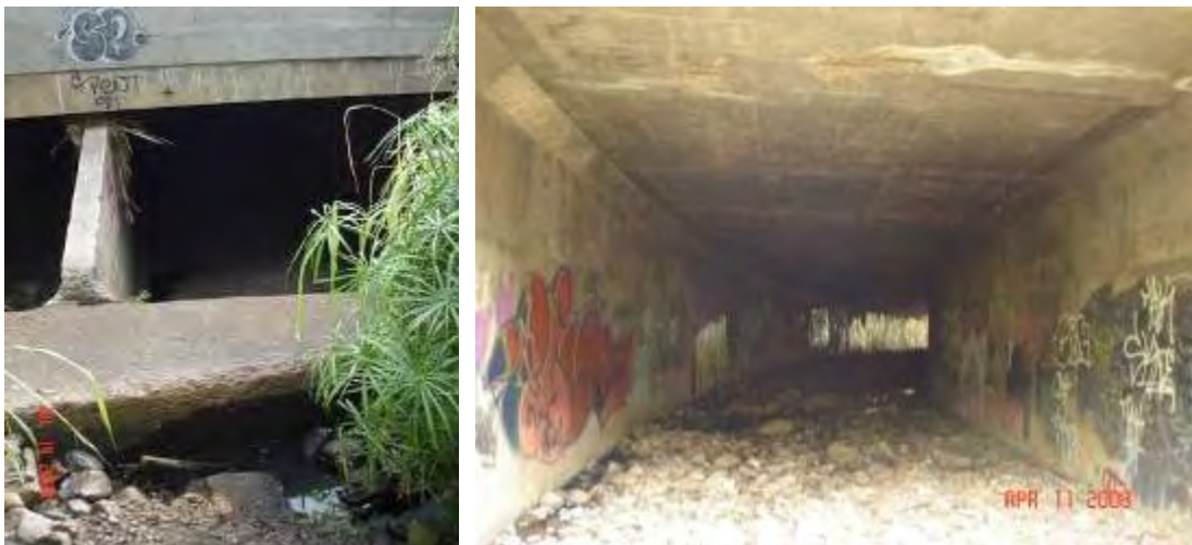
Figure 7. H-1 Freeway Culvert Inlet and Interior View.
