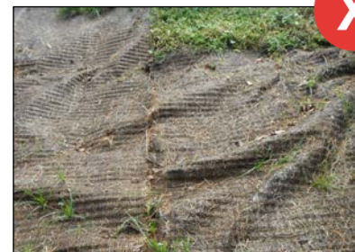
Matting must maintain direct contact with soil to prevent rills, gullies, and undermining.
