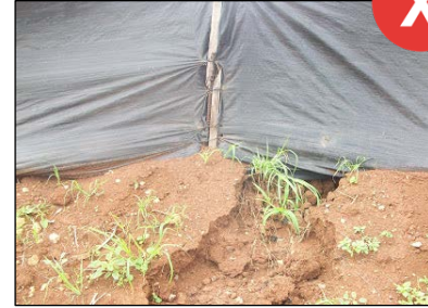
Repair or reinstall silt fence where undercutting has occurred.
