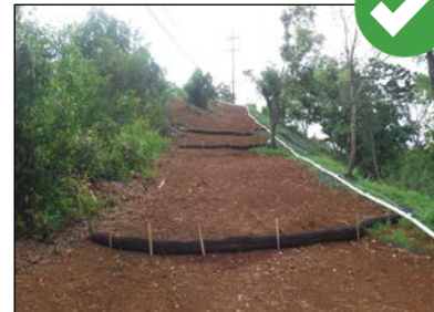
Compost filter berms must be staked into the slope to secure them into the ground.
