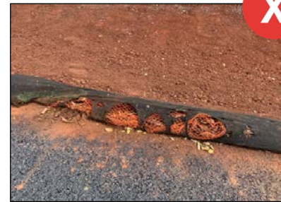
Repair/replace split, torn, or slumping compost filter socks to preserve filtration capabilities.
