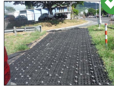
Alternative commercial construction entrance/exit products may be used if approved by the Engineer and installed per manufacturer's specifications.
