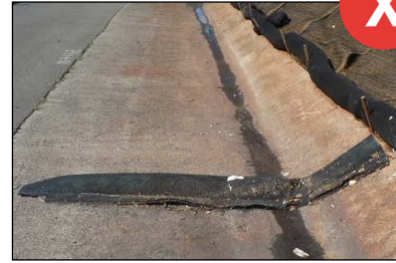
Check dams that get flattened must be repaired/replaced.
