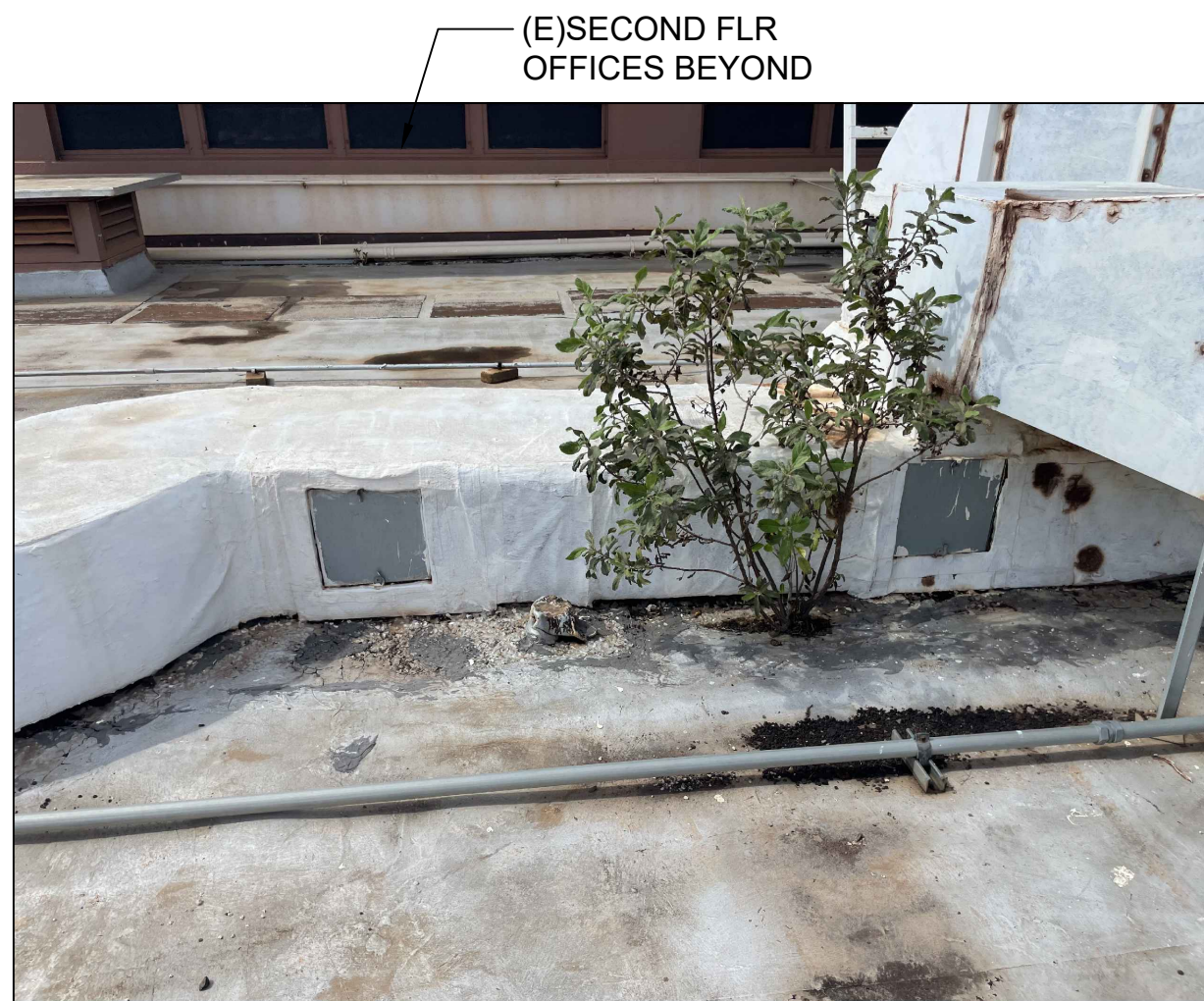
EXISTING ROOF PHOTOS
