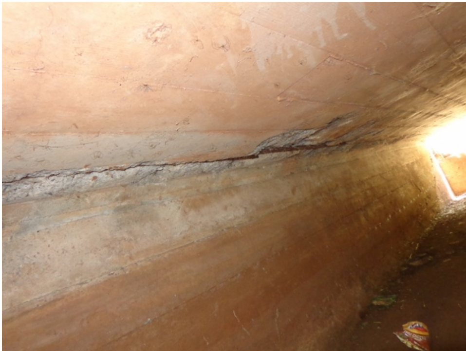
Photo 18: Spall measuring 10' long x 30" wide x 2" deep with 8 exposed reinforcing bars occurring in culvert soffit near outlet above the east culvert wall
