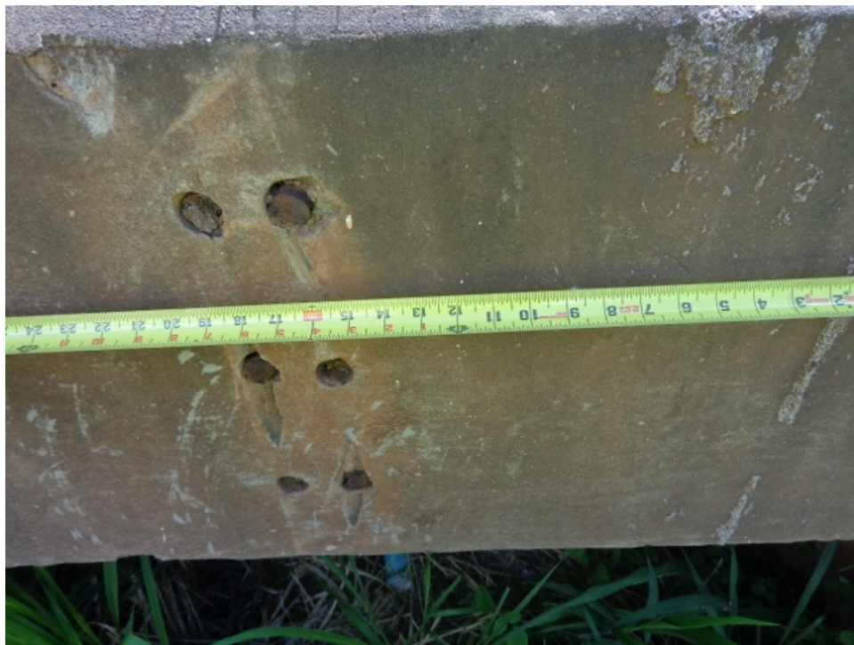
Photo 14: Corroded upstream guardrail posts embeddings in upstream headwall
