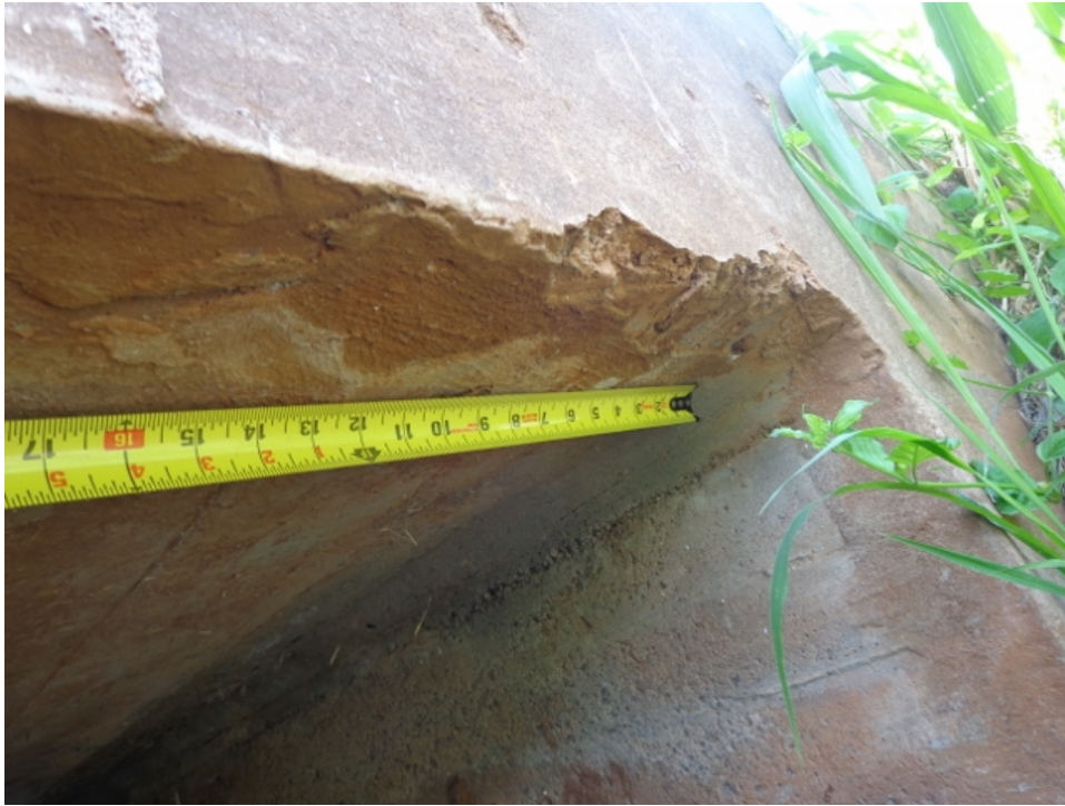
Photo 17: 12" long x 72" wide area of delamination occurring in culvert soffit at inlet
