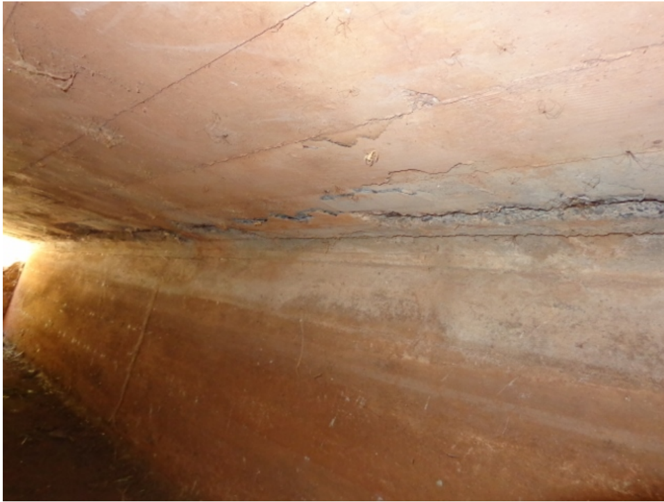
Photo 19: Spall measuring 10' long x 24" wide x 2" deep with 8 exposed reinforcing bars occurring in culvert soffit near outlet above the west culvert wall
