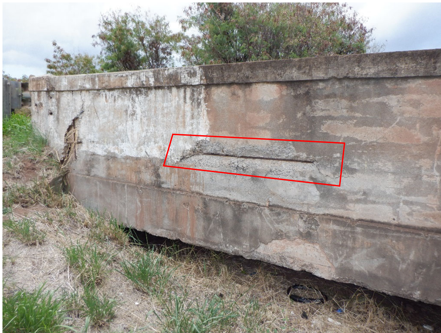
PHOTO 12 5'-3"X1'-6"X3" SPALL WITH EXPOSED REBAR (6FT 1080 CS3) ON EXTERIOR FACE OF UPSTREAM RAILING, 10' FROM NORTH END OF BRIDGE
