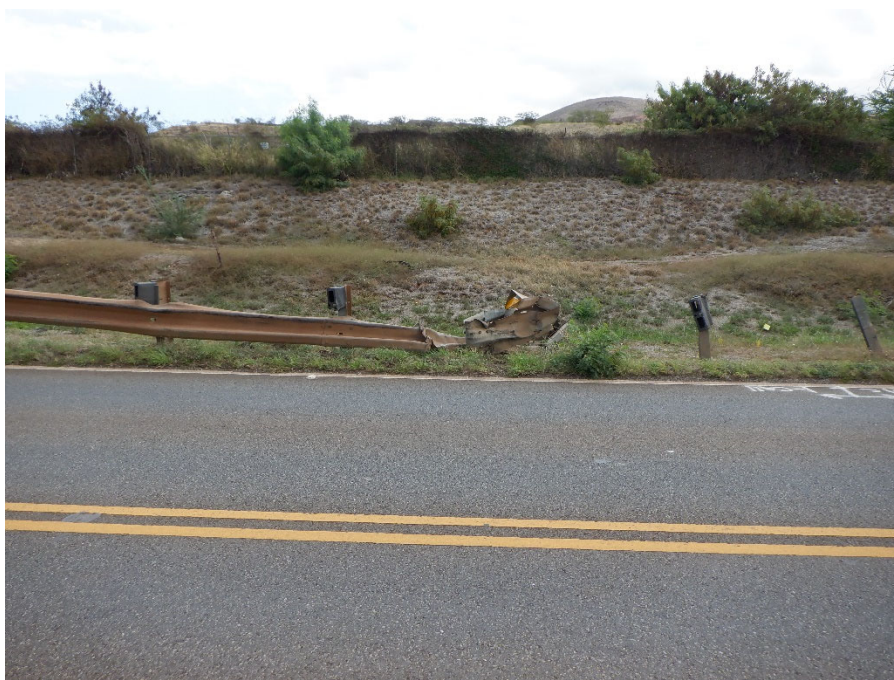
PHOTO 9 COLLISION DAMAGE TO UPSTREAM NORTH APPROACH GUARDRAIL AND END TREATMENT
