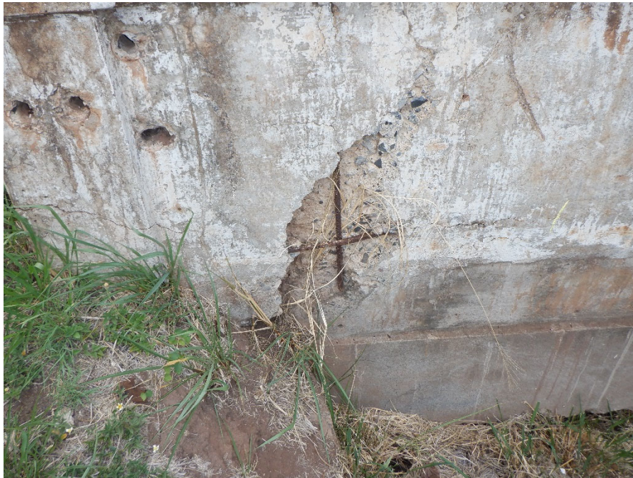
PHOTO 10 3'X3'X4" SPALL WITH EXPOSED REBAR (3FT 1080 CS3) ON EXTERIOR FACE OF UPSTREAM RAILING, 2' FROM NORTH END OF BRIDGE
