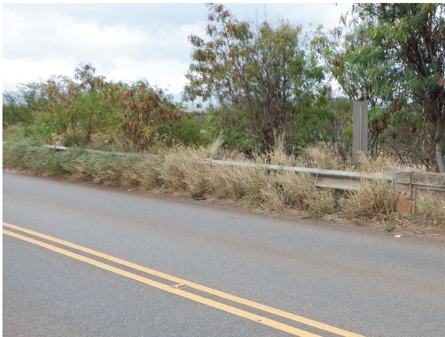
PHOTO 8 DOWNSTREAM NORTH APPROACH GUARDRAIL WITH VEGETATION
