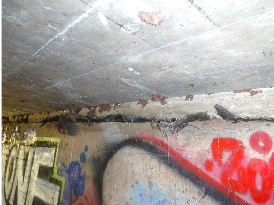
PHOTO 19 PROTRUDING ROOFING PAPER ALONG TOP OF ABUTMENT 1
