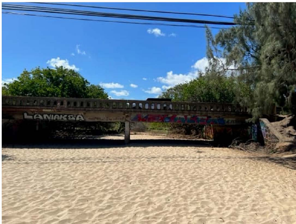
View of existing bridge from beach.
