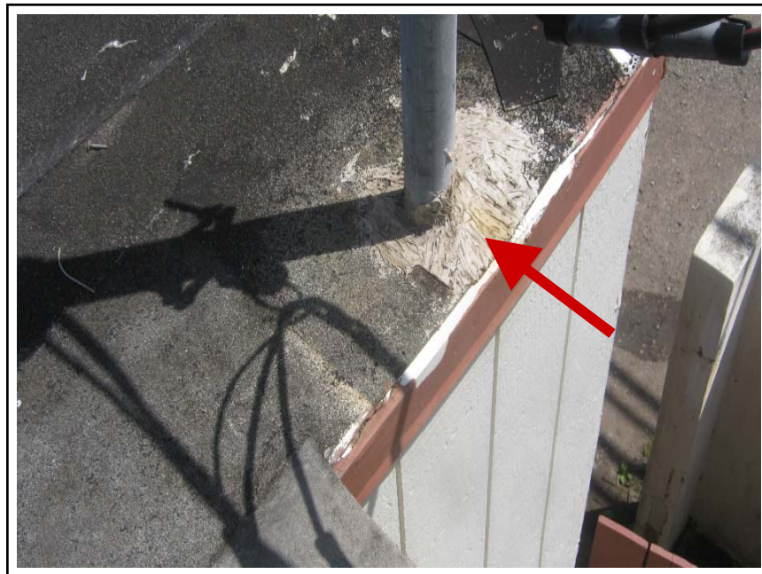
1907-003B-A19: White Caulking on Pipe Penetration with Black Mastic Building B Studio Roof
