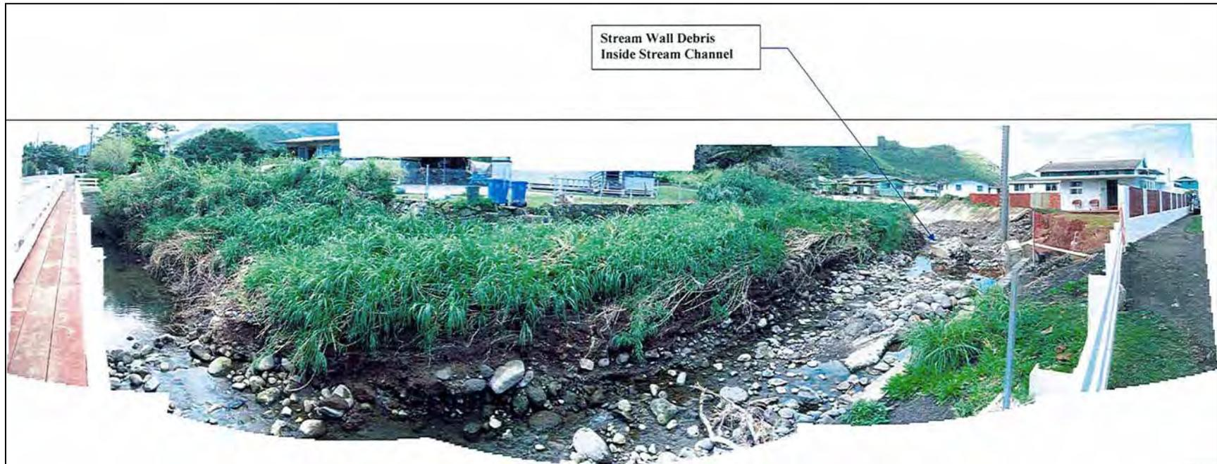
Figure 5. Panorama view upstream of Kaipapa‘u Stream Bridge showing location of failed stream wall (at right)
