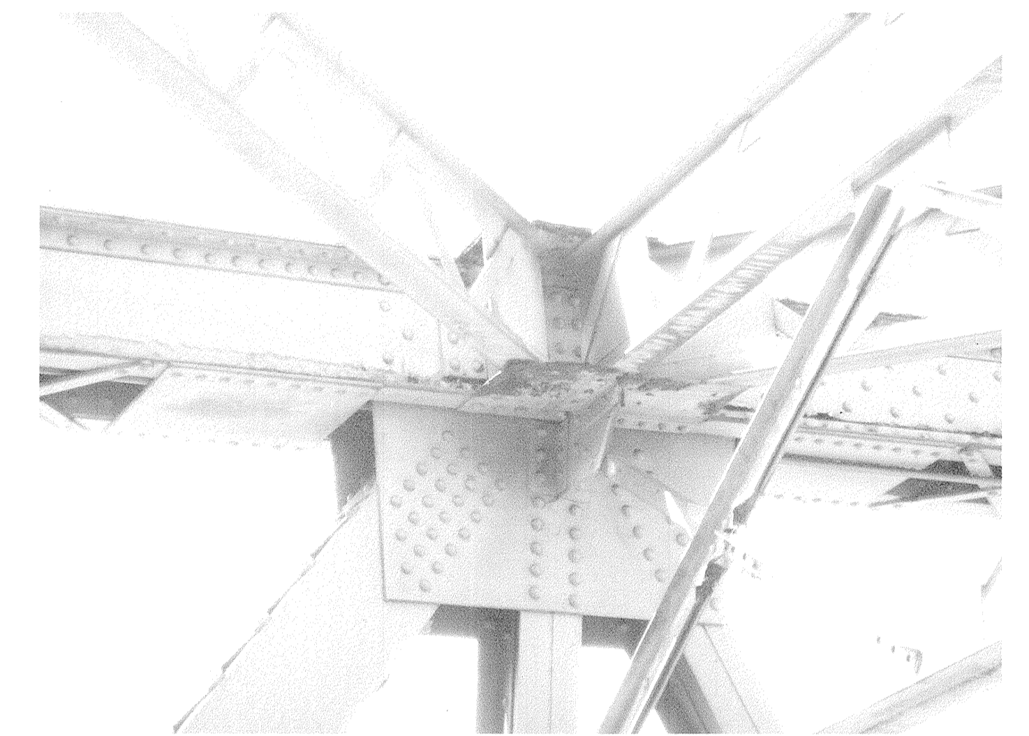
2 PHOTO - EXAMPLE GUSSET PLATE CONN S4.6 | S4.6 (TYPE 2 SHOWN)
