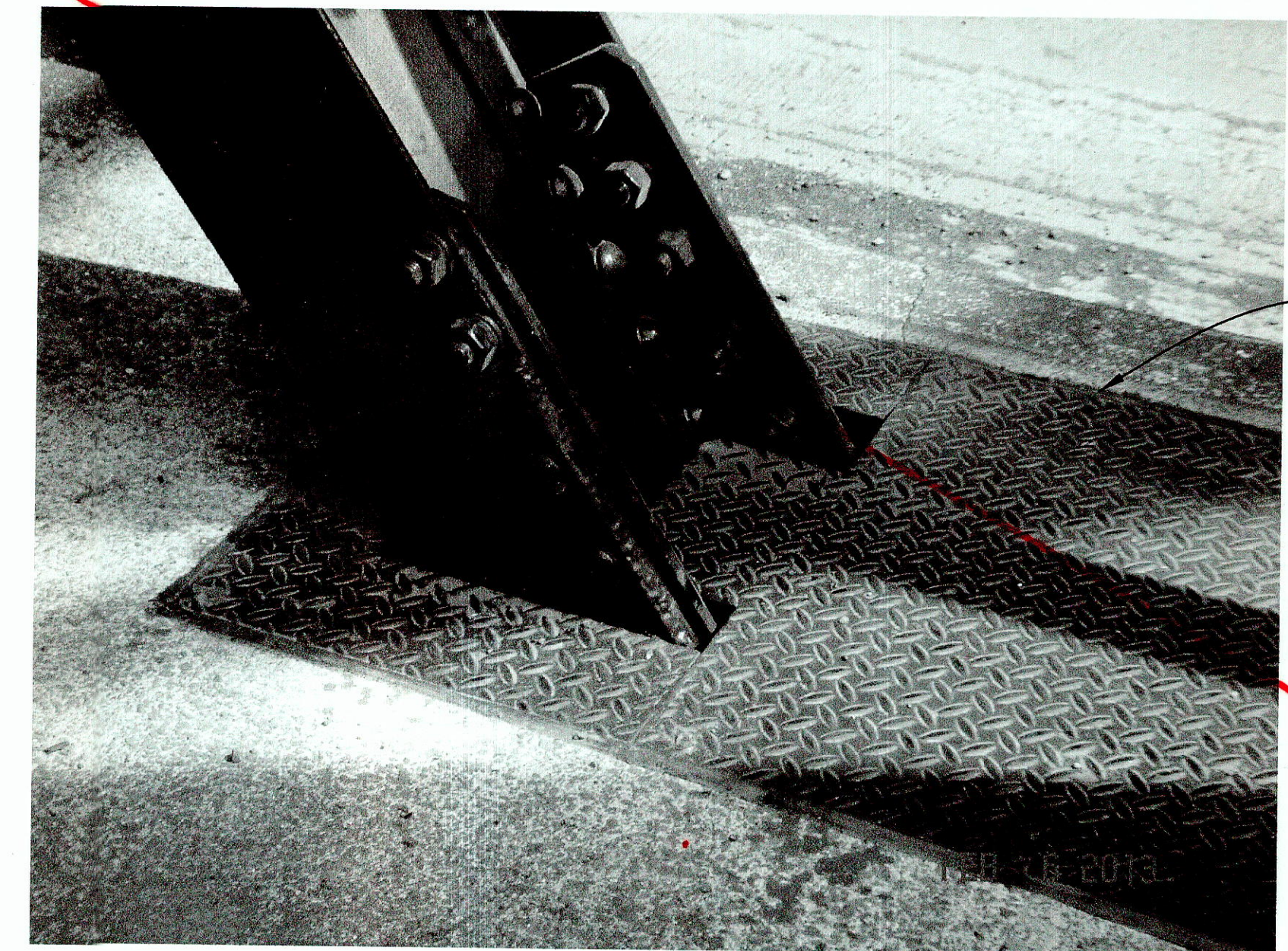
3 PHOTO - COVER PLATE AT DECK OPENING S7.8, S9.1, S7.8
