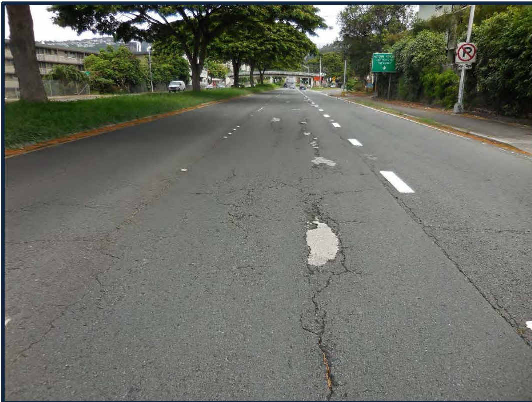
Photo No. 2: Concrete pothole patching along longitudinal cracks.
