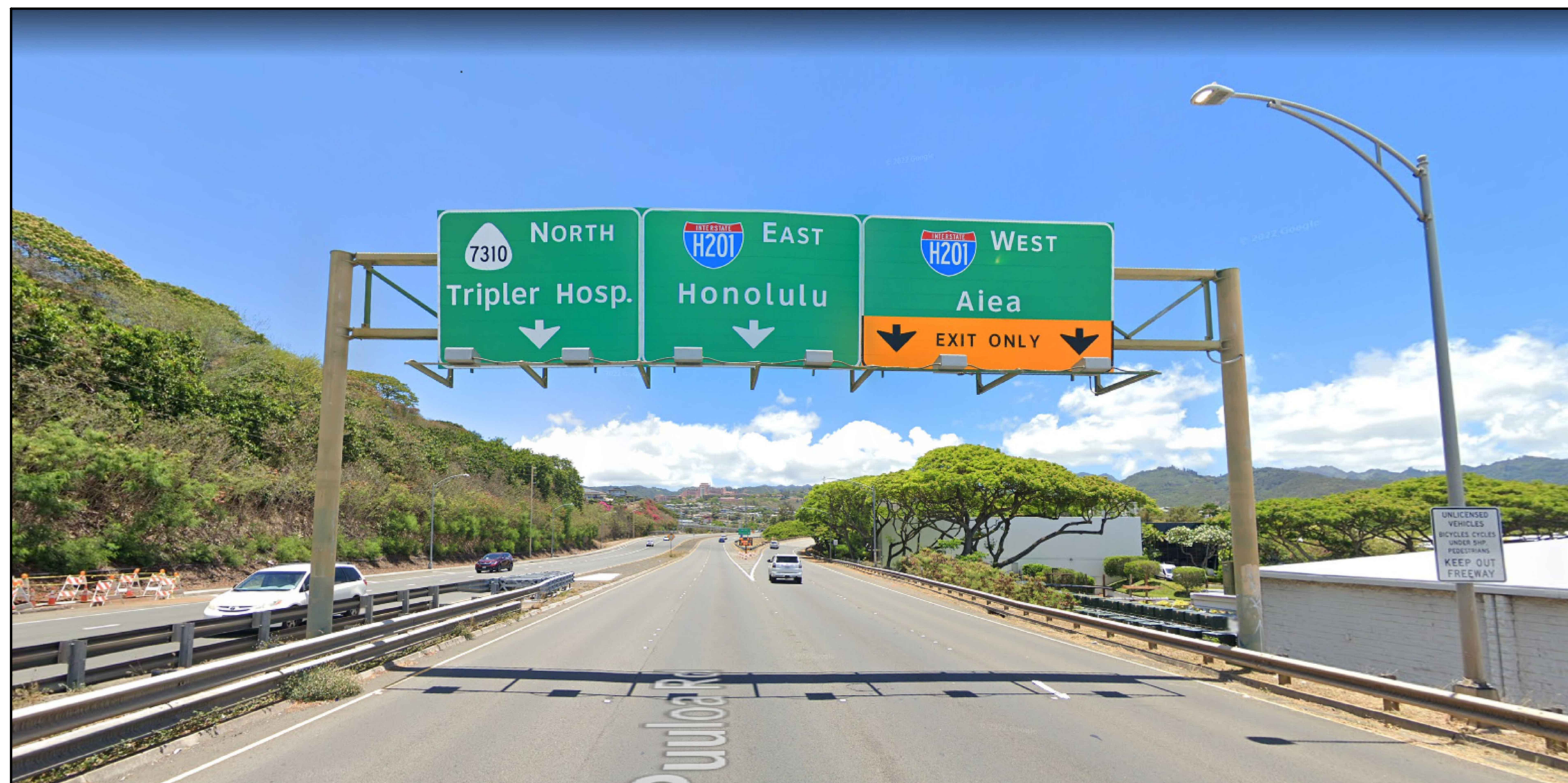
EXISTING SIGN STRUCTURE H201R-874
