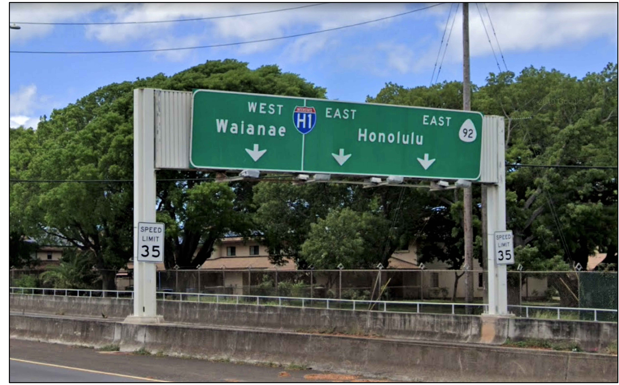
EXISTING SIGN STRUCTURE HIEBR-260
