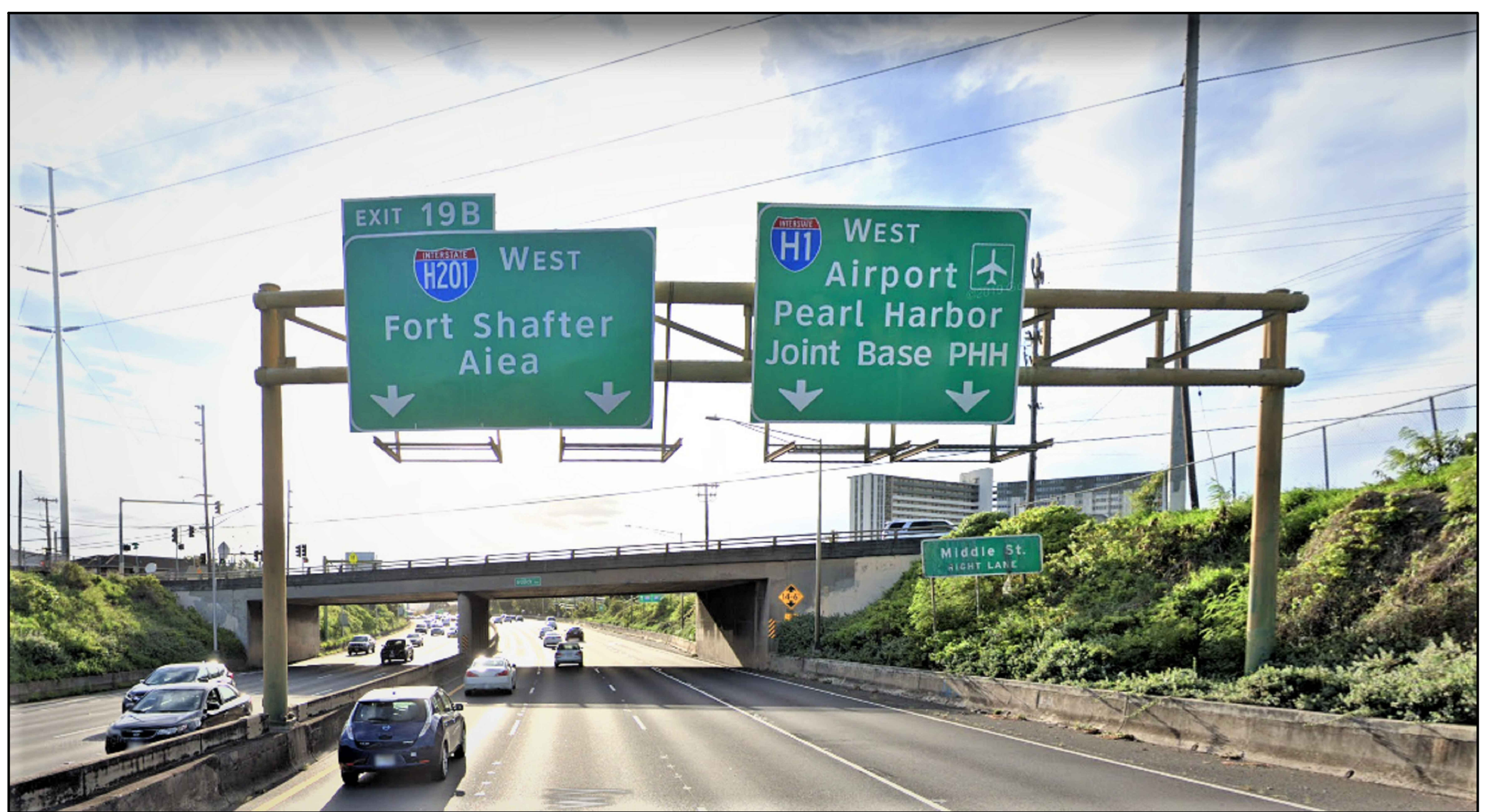
EXISTING SIGN STRUCTURE H1WB-421
