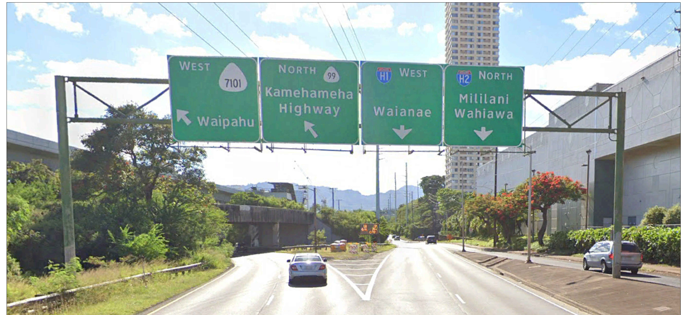
EXISTING SIGN STRUCTURE H2NBR-722
