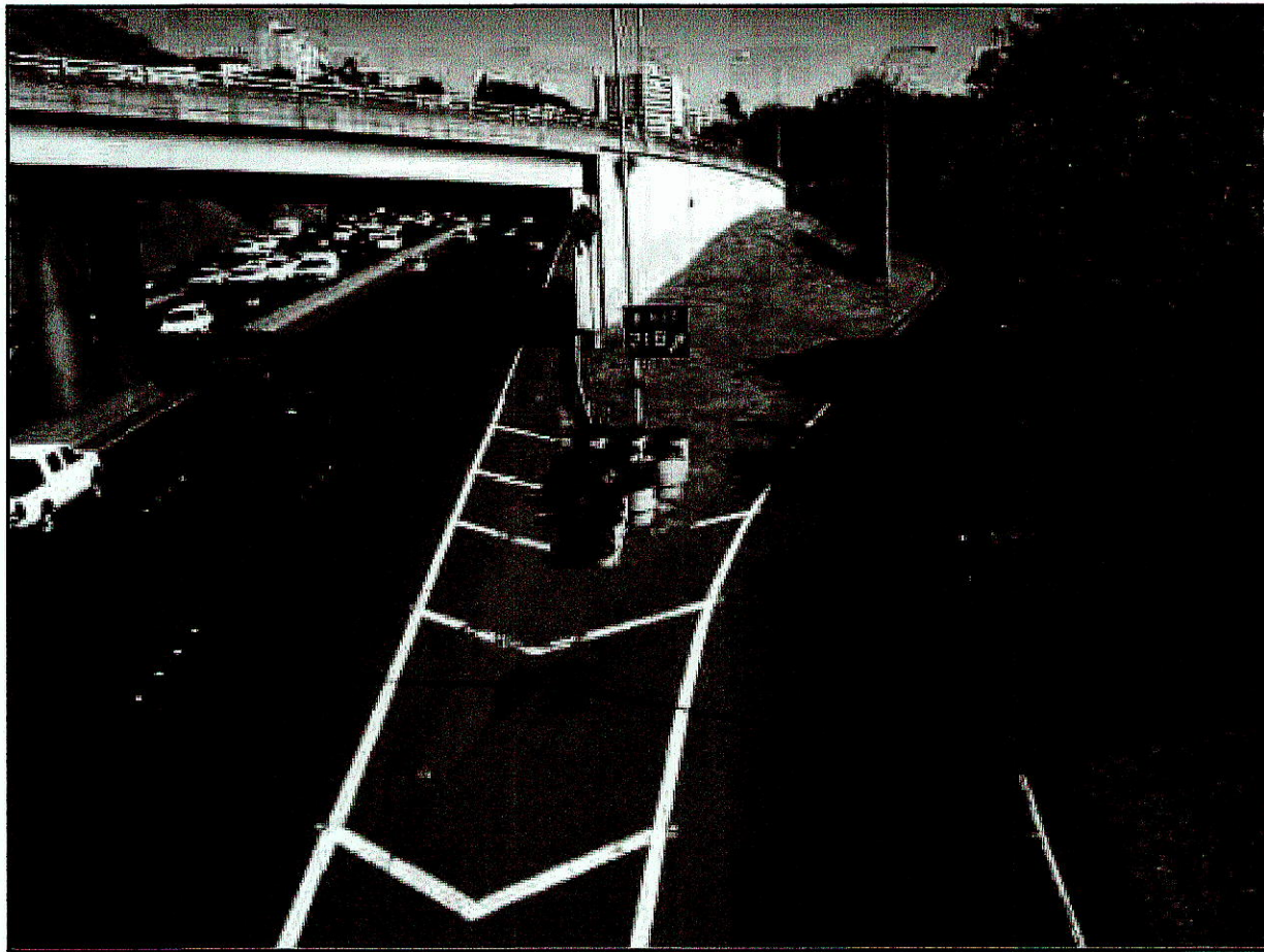
PICTURE 1 EASTBOUND TRAFFIC N.T.S.
