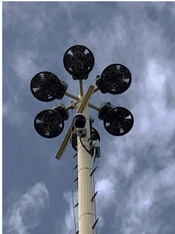
Photo 10: Matson-Owned Camera and Transceiver at Light Pole 53-19
