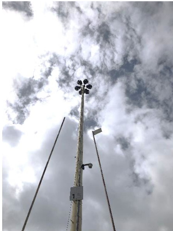
Photo 2: Light Pole 53-3 with Matson-Owned Container Tracking System and Transceiver
