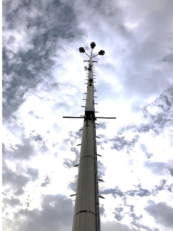
Photo 5: Light Pole 53-8 with Matson-Owned Antenna, Junction Box, Security Camera, and Transceiver
