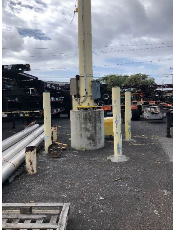
Photo 9: Light Pole 53-19 with Panelboard and Matson-Owned Telecommunications Cabinet
