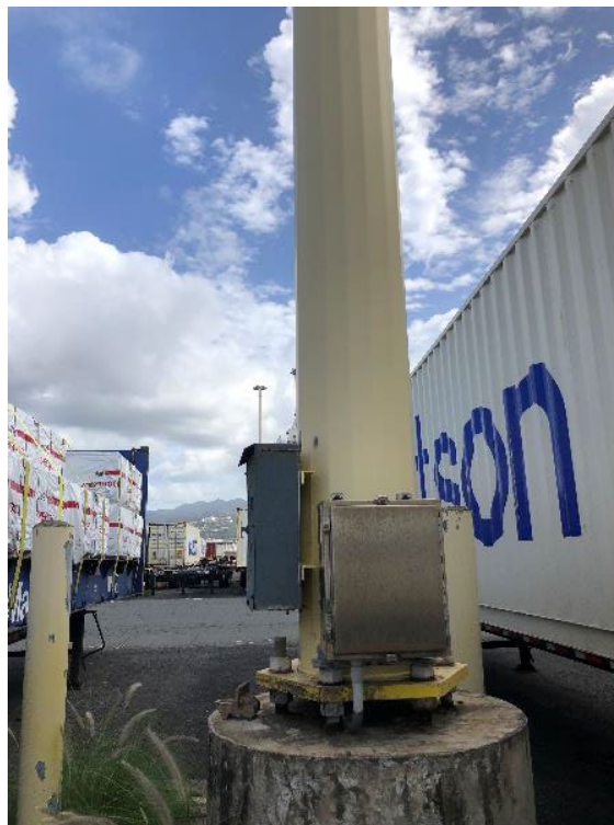
Photo 6: Light Pole 53-14 with Panelboard and Matson-Owned Fiber Splice Box
