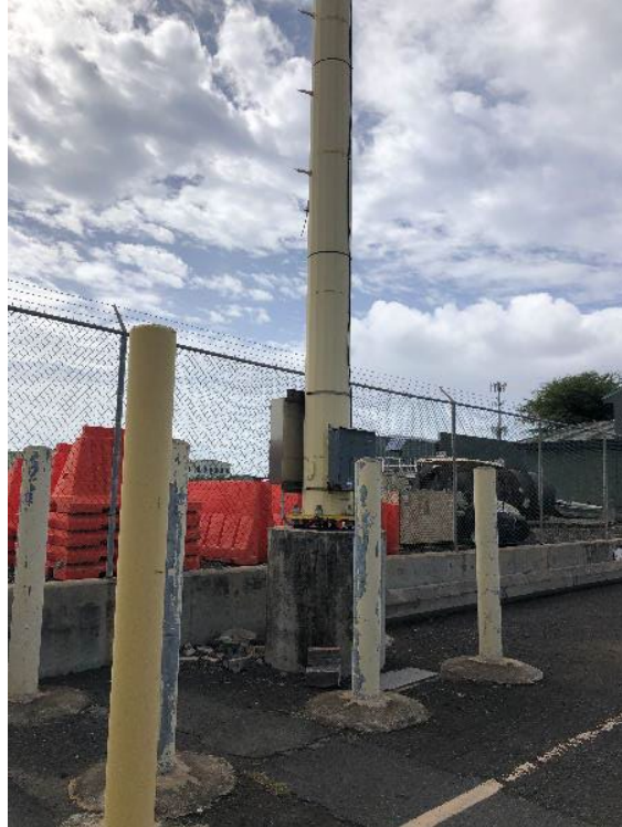
Photo 7: Light Pole 53-15 with Panelboard and Matson-Owned Telecommunications Cabinet
