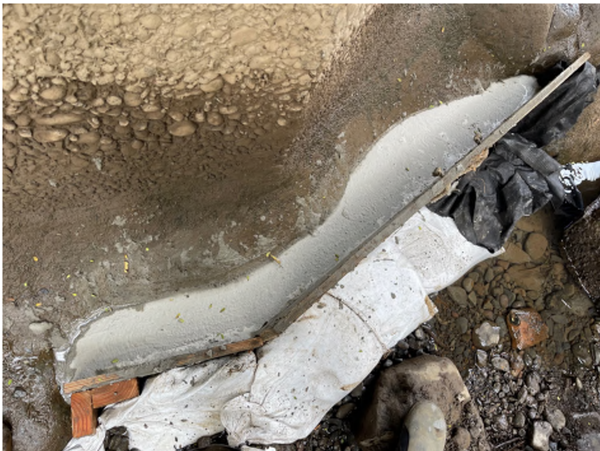
Poured In Place Segment 22" L x 8" H x 8" D
