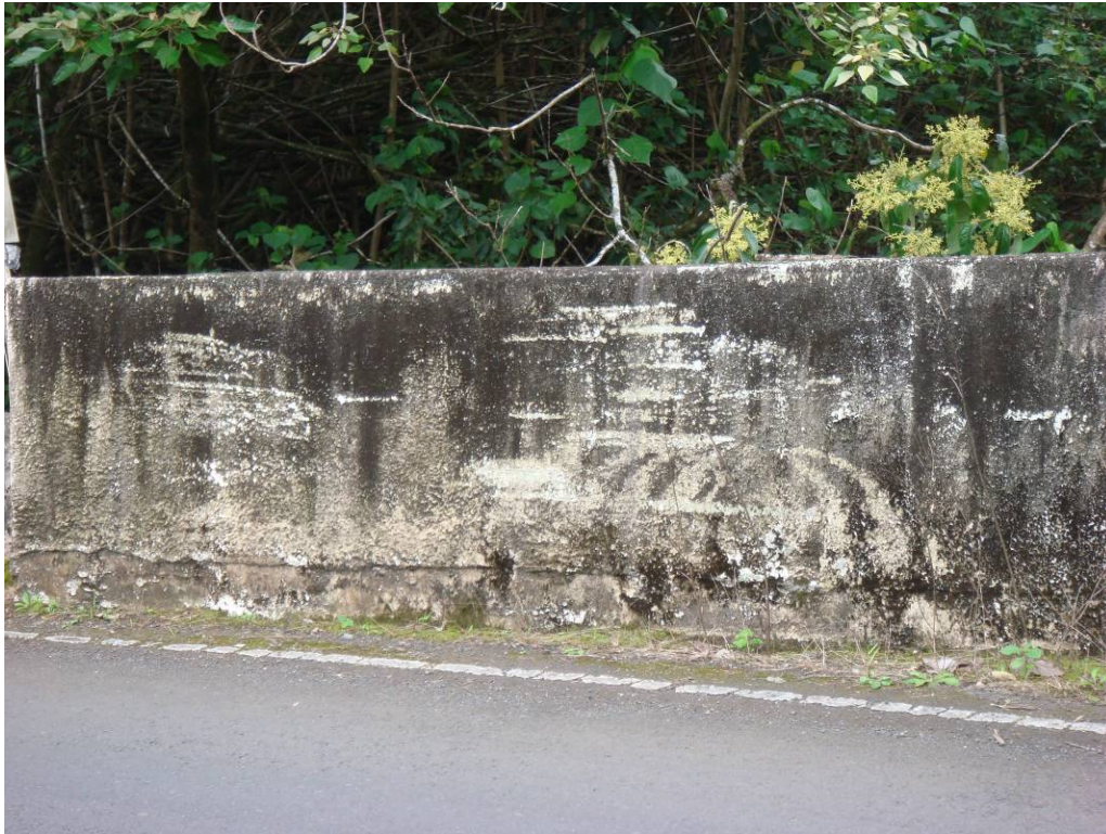
PHOTO 9 CLOSE UP OF SCRAPES ON UPSTREAM PARAPET NEAR HANA SIDE
