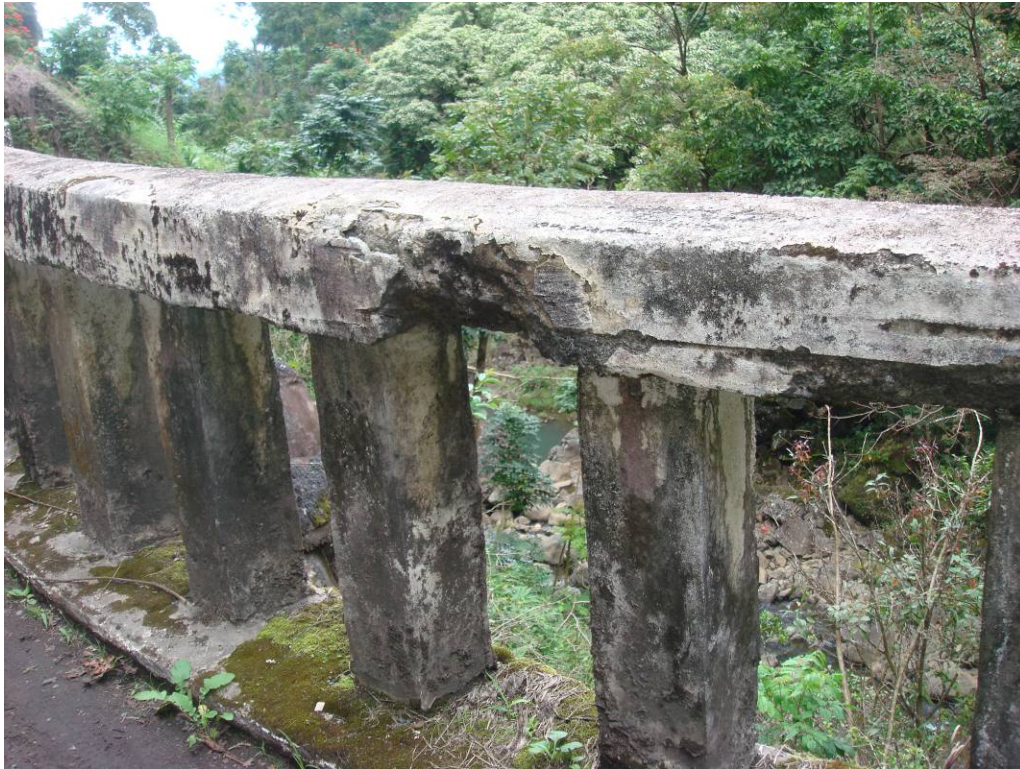
PHOTO 13 CLOSE UP OF SPALL WITH EXPOSED REBAR IN DOWNSTREAM RAILING CAP
