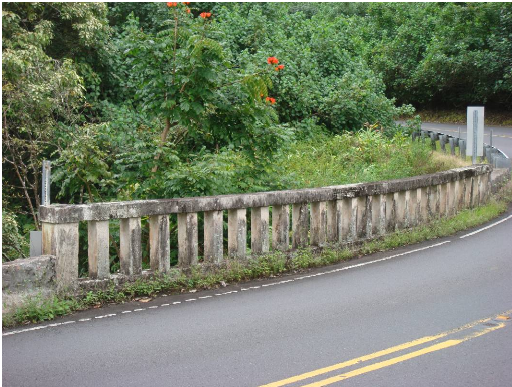
PHOTO 10 DOWNSTREAM RAILING ELEVATION. NOTE: RAILING HT = 40"
