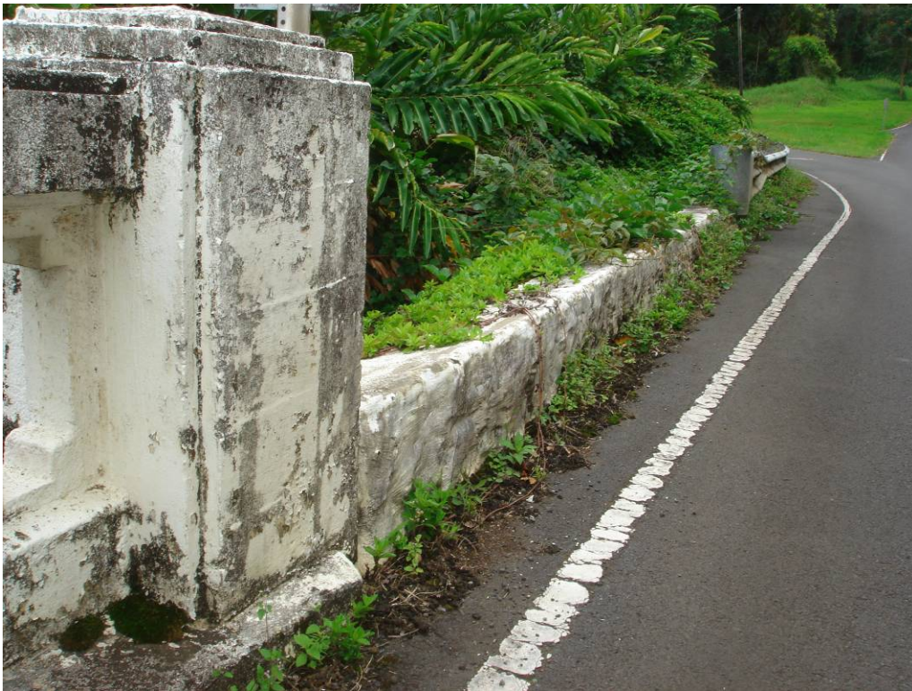
PHOTO 8 DOWNSTREAM HANA CRM WALL
