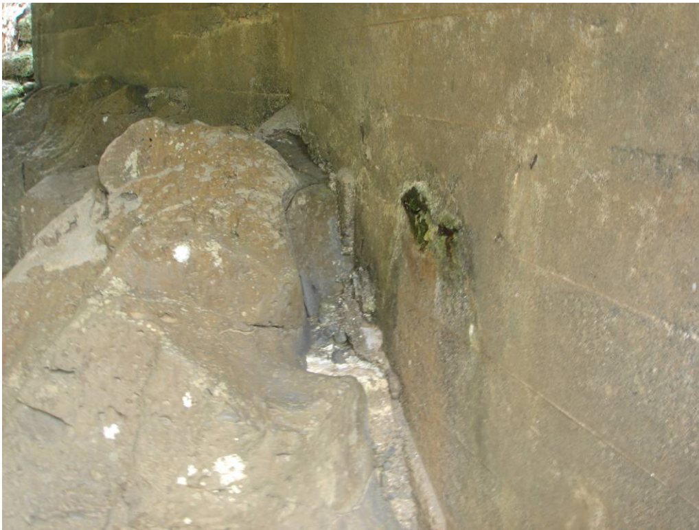
PHOTO 30 SPALL IN KAHULUI ABUTMENT UNDER GIRDERS G4 AND G5
