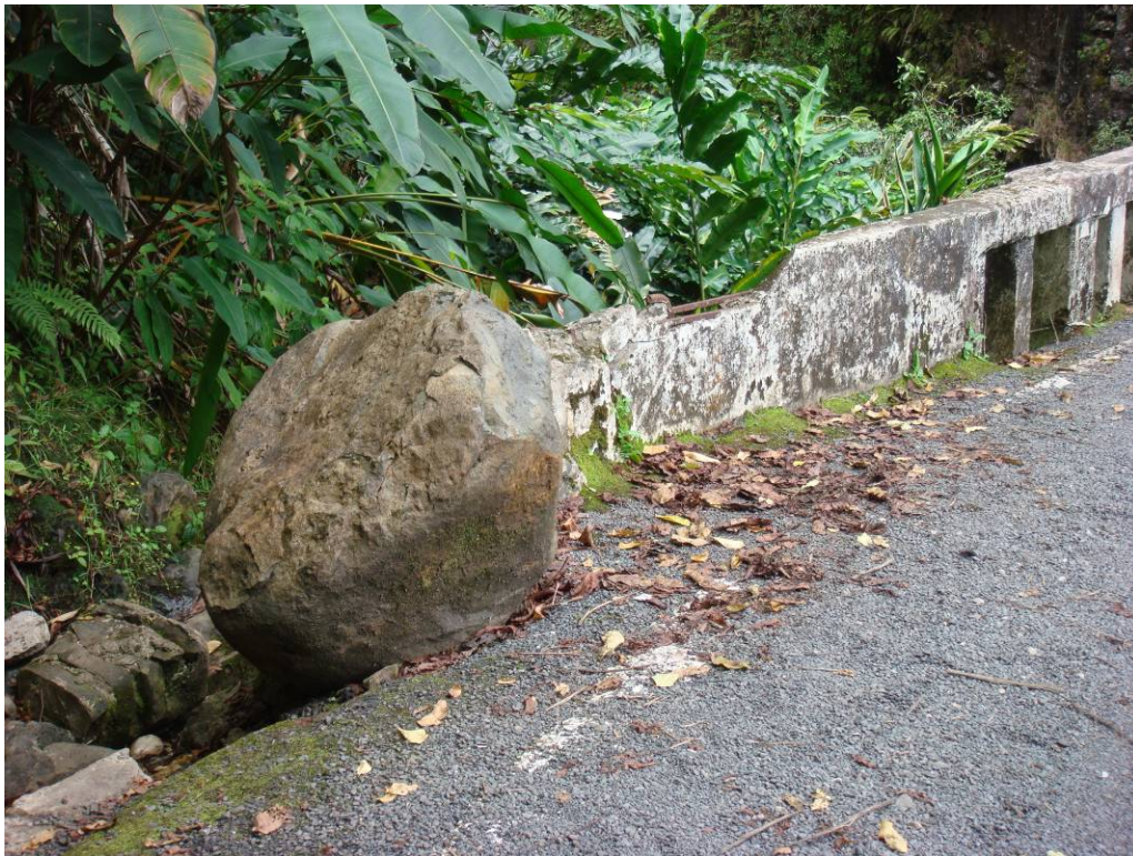
PHOTO 6 UPSTREAM / HANA CONCRETE PARAPET WITH COLLISION DAMAGE AND EXPOSED REBAR. NOTE: PARAPET HEIGHT VARIES DUE TO COLLISION DAMAGE
