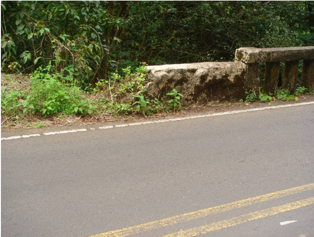
PHOTO 5 DAMAGE TO END OF DOWNSTREAM KAHULUI CRM WALL
