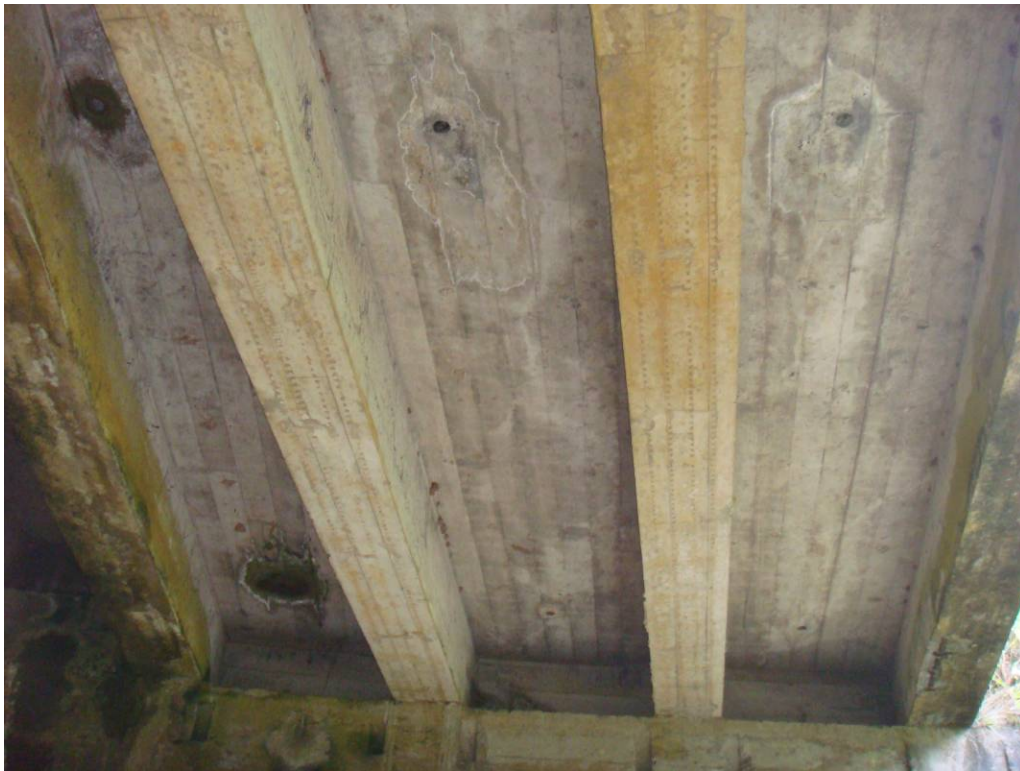
PHOTO 14 DOWNSTREAM HALF OF SOFFIT LOOKING TOWARD KAHULUI WITH EFFLORESCENCE AND WATER STAINS. NOTE: DECK DRAINS HAVE BEEN PAVED OVER
