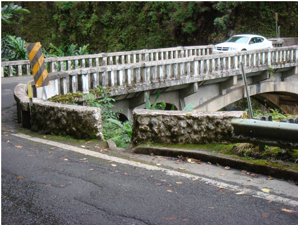
PHOTO 8 DOWNSTREAM / HANA GUARDRAIL AND CRM WALL. NOTE: GUARDRAIL HT = 27"
