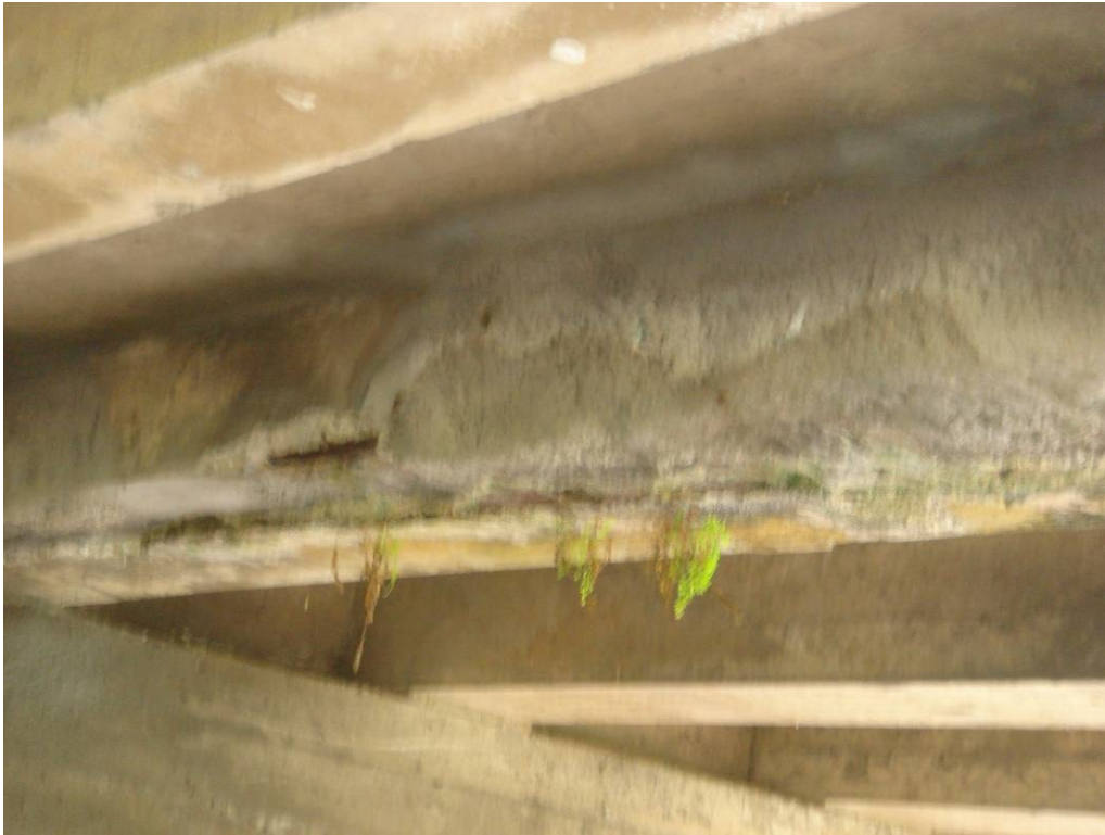
PHOTO 19 SPALL WITH EXPOSED REBAR AND UNSOUND PATCH IN GIRDER G4
