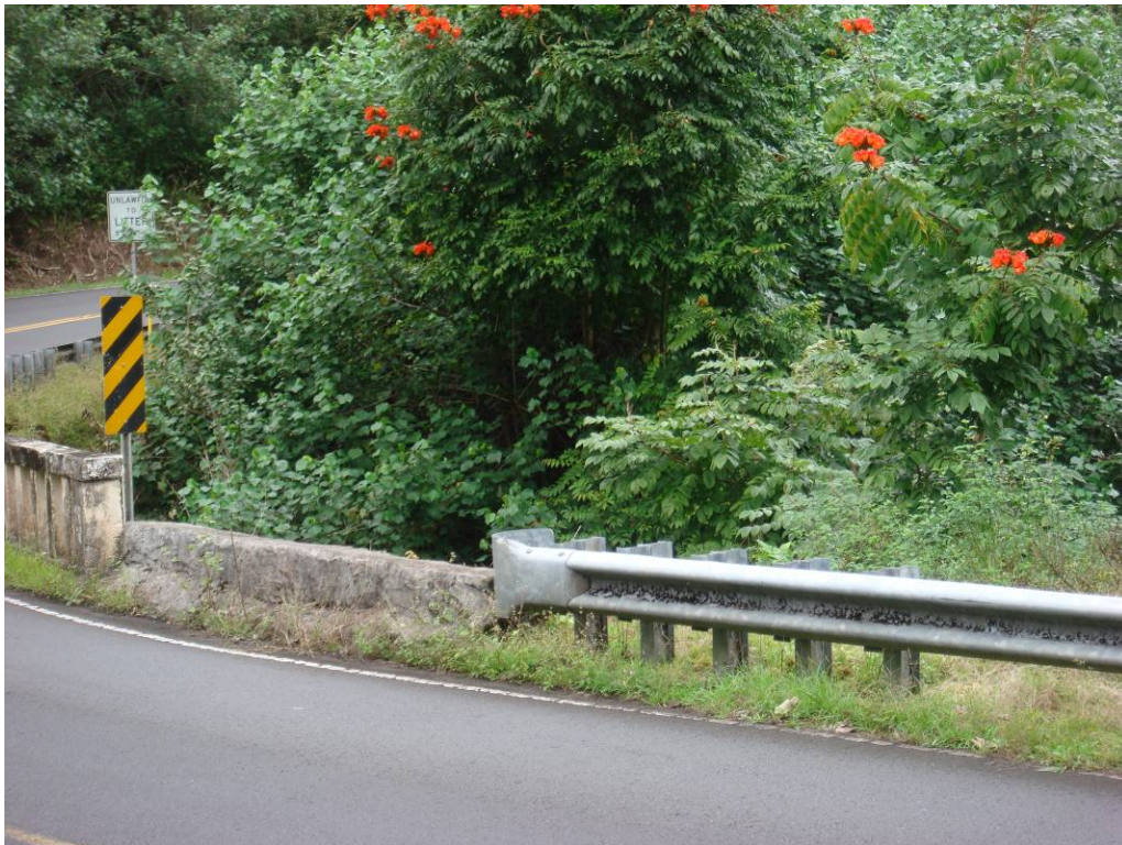
PHOTO 6 DOWNSTREAM / HANA GUARDRAIL END TREATMENT AND CRM WALL. NOTE: GUARDRAIL END TREATMENT HT = 26"
