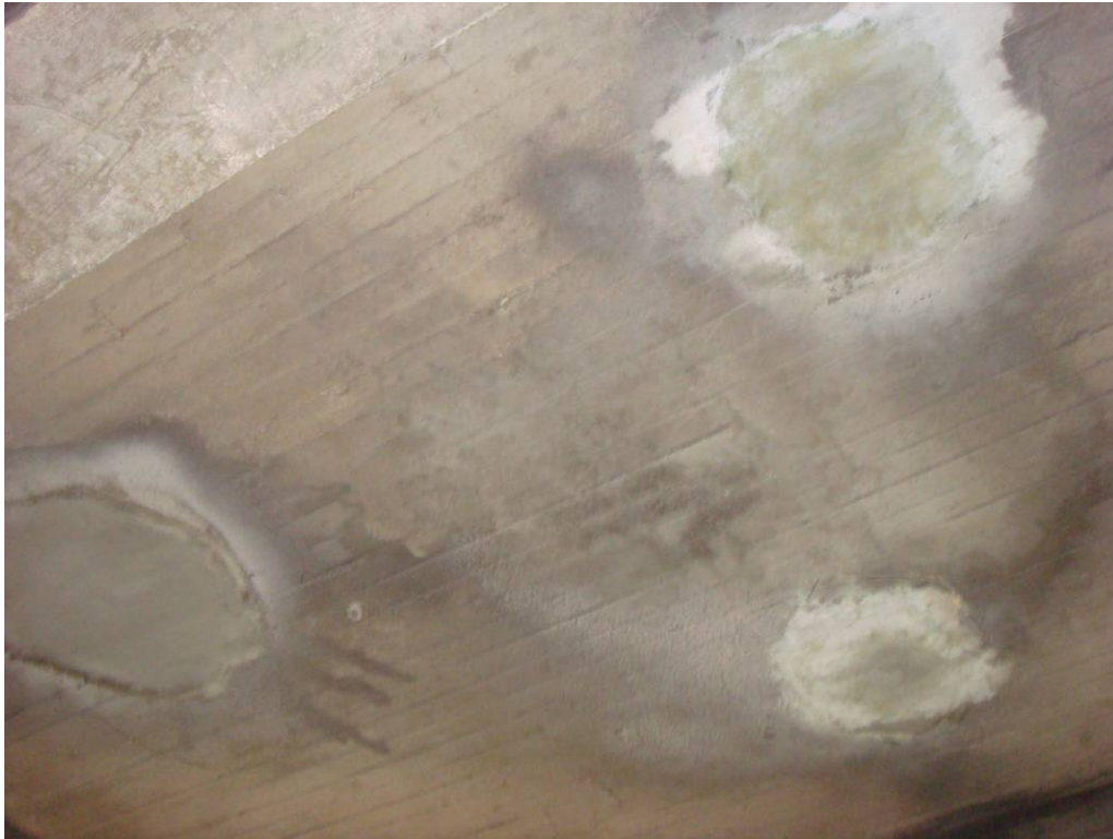
PHOTO 25 PATCHES IN SOFFIT BETWEEN SPANDREL BENT 1 AND 2. NOTE: SPANDREL COUNT STARTS FROM HANA ABUTMENT.
