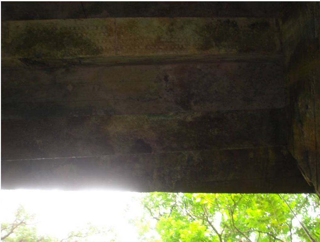
PHOTO 16 HONEYCOMBING IN CANTELEIVERED SOFFIT UPSTREAM END
