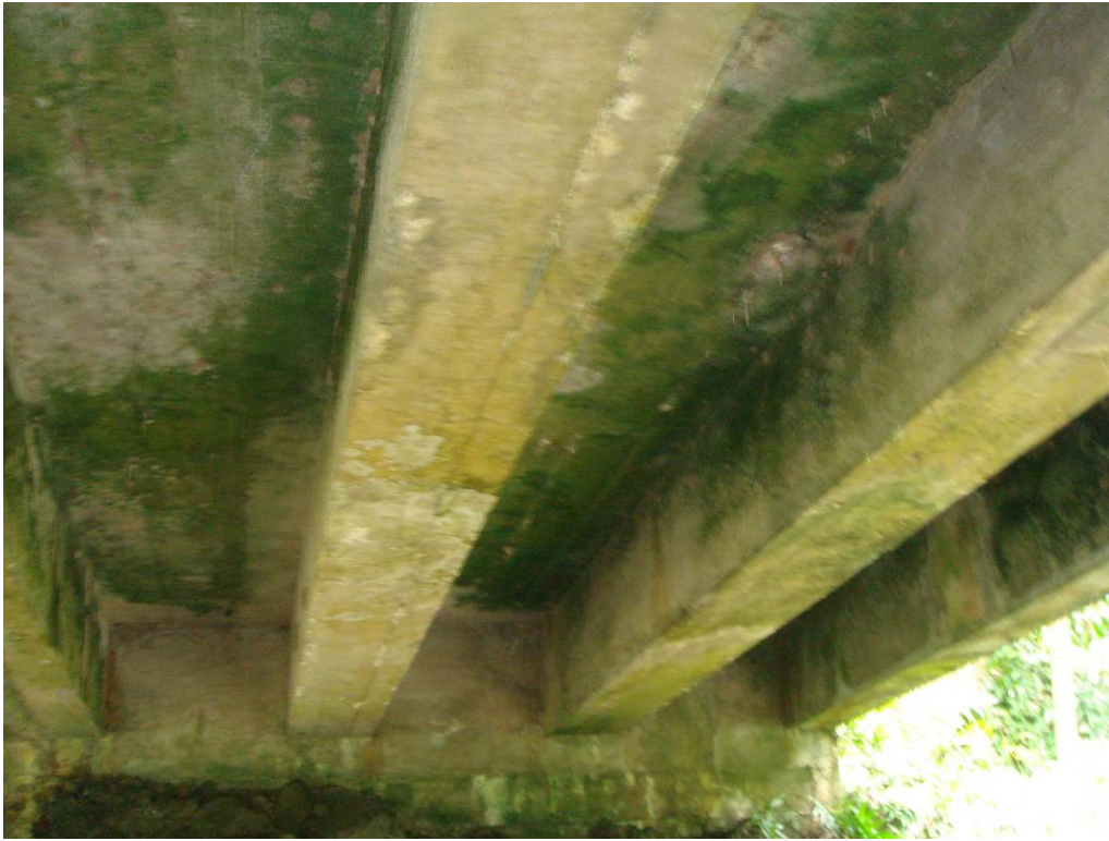
PHOTO 15 DOWNSTREAM HALF OF SOFFIT LOOKING TOWARD KAHULUI WITH EFFLORESCENCE AND MOSS. DELAMINATION IN GIRDER G6 DOWNSTREAM FACE NEAR KAHULUI ABUTMENT.
