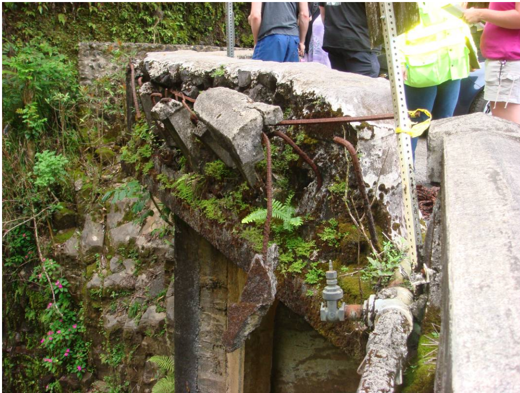
PHOTO 4 COLLISION DAMAGE WITH EXPOSED REBAR AT FORMER CONCRETE BRIDGE RAILING AT UPSTREAM / KAHULUI SIDE
