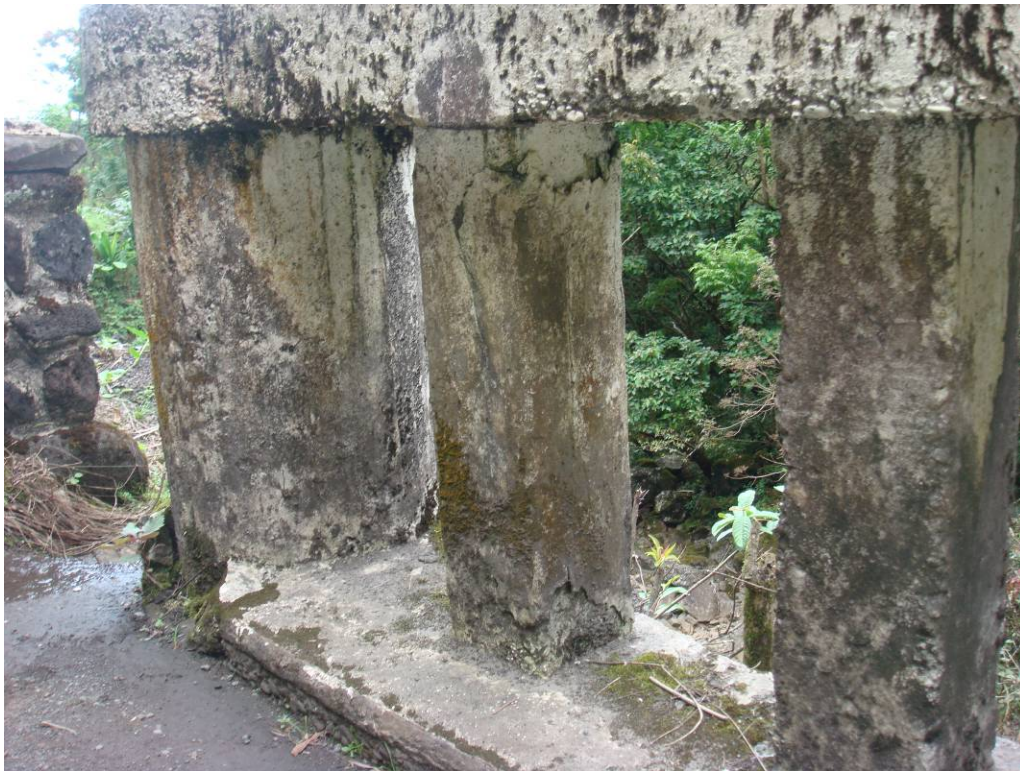
PHOTO 14 DELAMINATION ON SECOND PICKET AT DOWNSTREAM / KAHULUI RAILING
