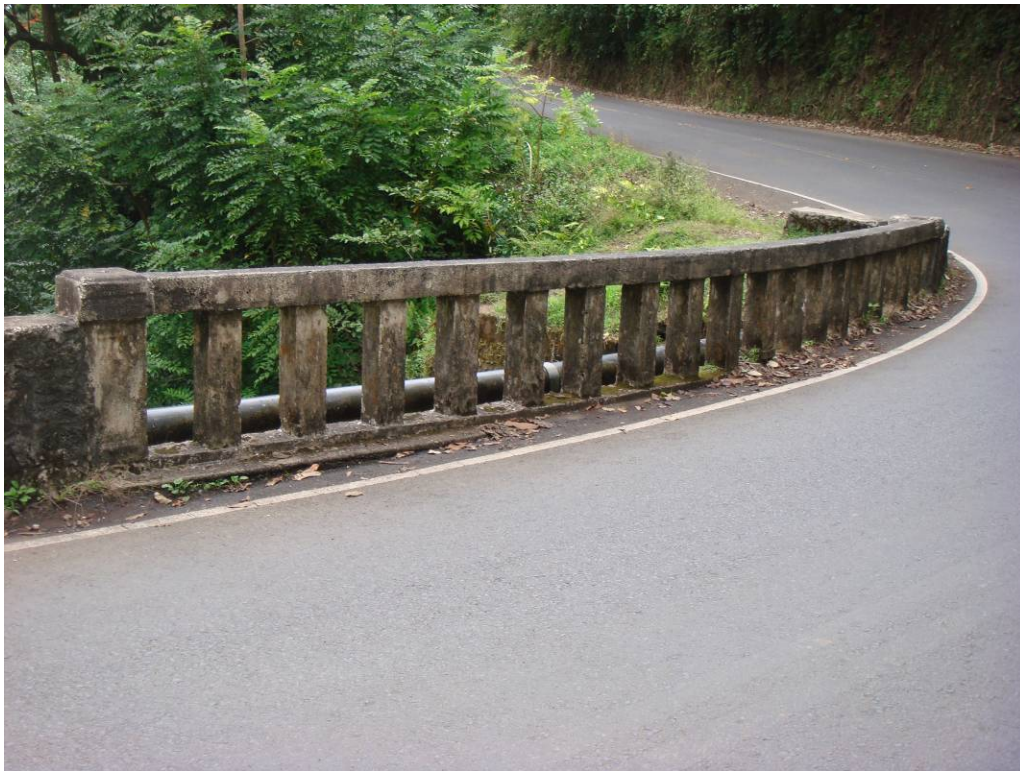
PHOTO 10 DOWNSTREAM BRIDGE RAILING. NOTE: RAILING HT = 33"
