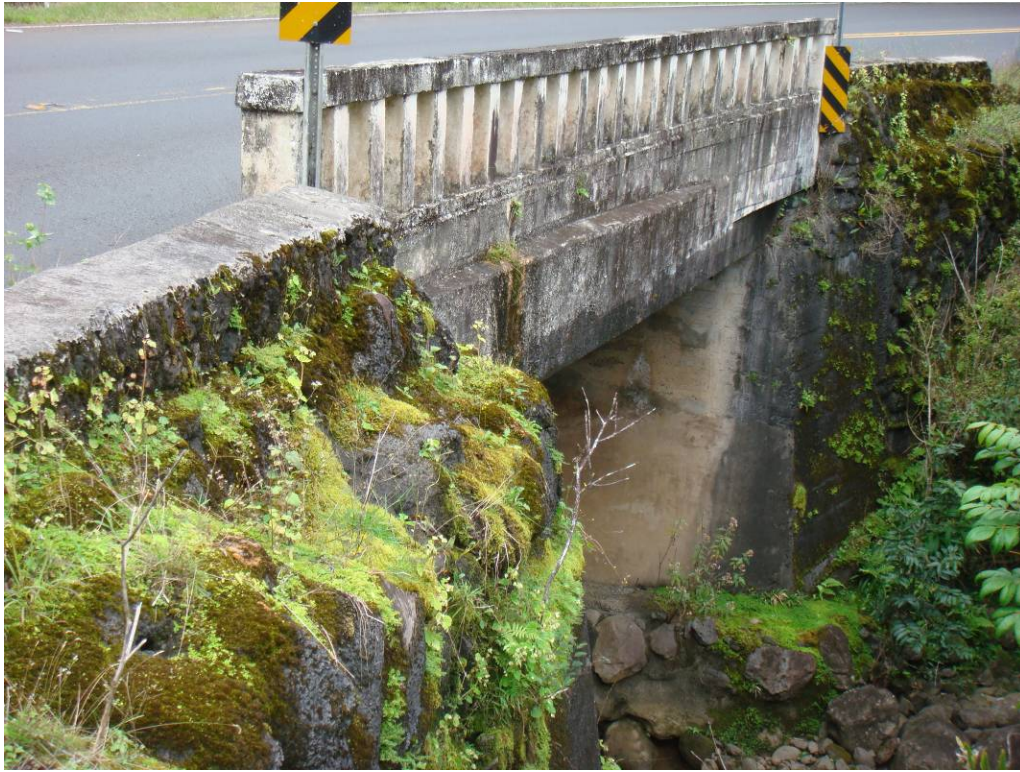
PHOTO 11 BACKSIDE DOWNSTREAM RAILING ELEVATION. NOTE: DAMAGED RM-4 SIGN AT THE KAHULUI END OF RAILING
