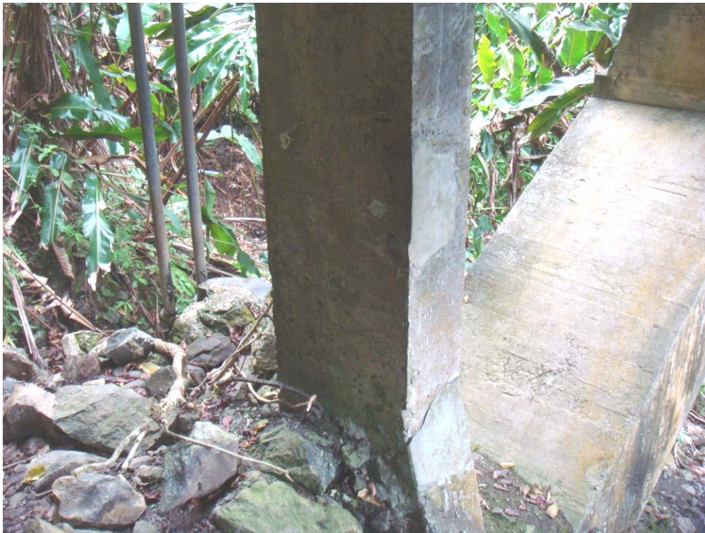
PHOTO 28 SMALL SPALL WITH EXPOSED REBAR ON HANA FACE OF UPSTREAM SPANDREL COLUMN IN SPANDREL BENT 1.
