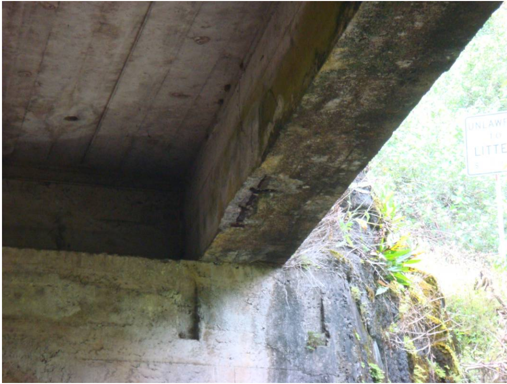
PHOTO 17 CLOSE UP OF LARGE SPALL WITH EXPOSED REBAR IN BOTTOM OF GIRDER G8 NEAR KAHULUI ABUTMENT
