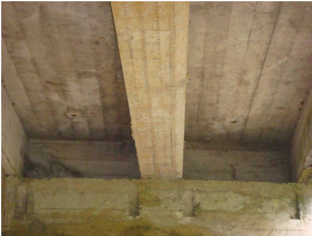
PHOTO 20 HONEYCOMBING BETWEEN GIRDERS G6 AND G7 AND DELAMINATION BETWEEN GIRDERS G7 AND G8 ON BACKWALL OF KAHULUI ABUTMENT
