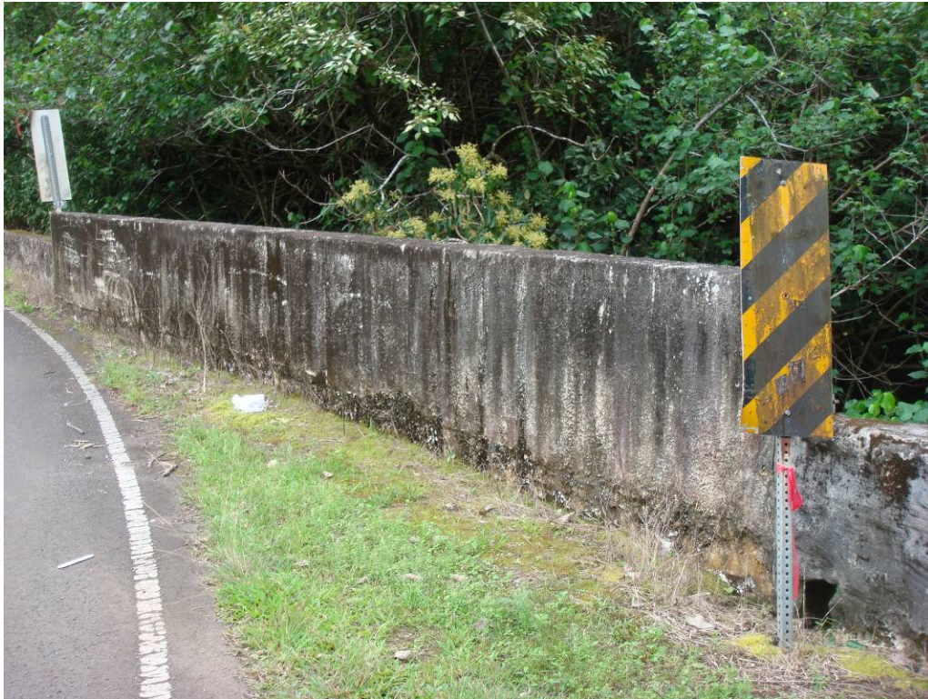
PHOTO 7 UPSTREAM PARAPET ELEVATION. NOTE: PARAPET HT = 42"
