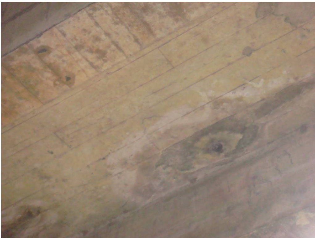
PHOTO 16 DELAMINATION IN DECK SOFFIT BETWEEN GIRDERS G3 AND G4 NEAR MID-SPAN
