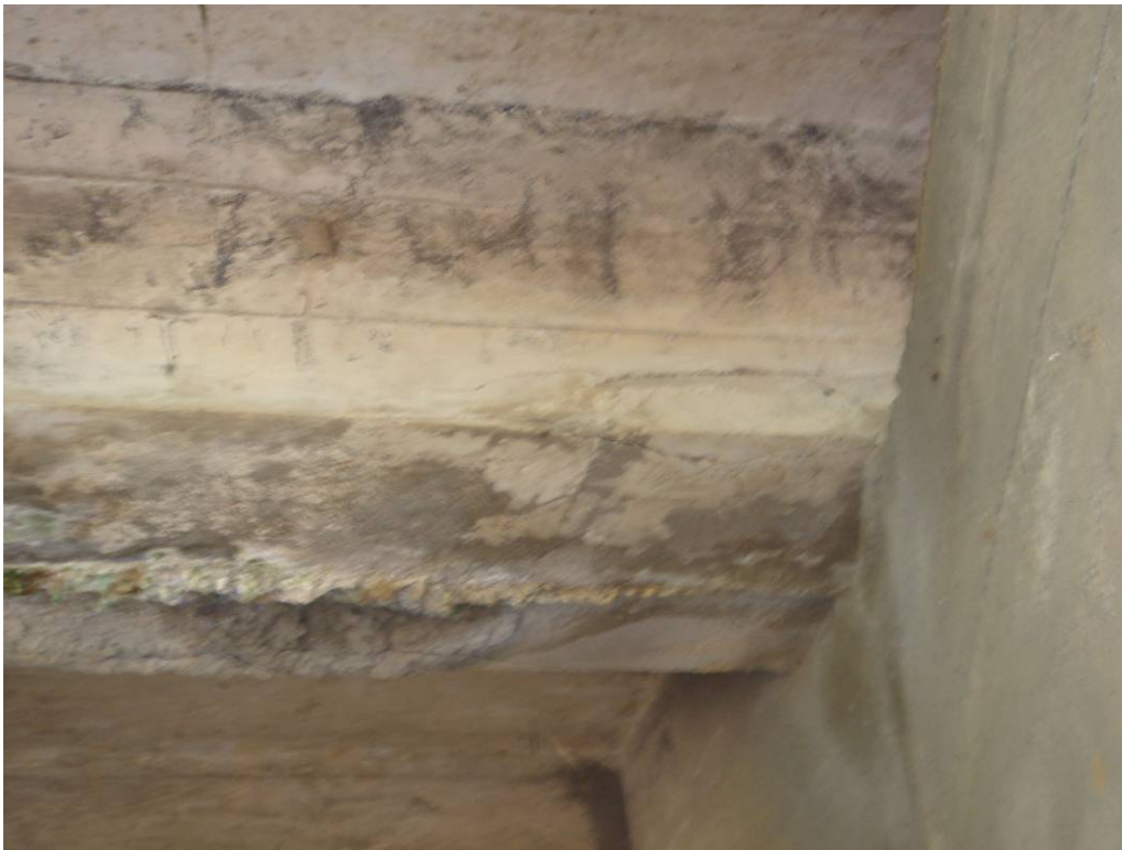
PHOTO 18 DELAMINATION AND UNSOUND PATCH IN GIRDERS G5 AND G6 NEAR KAHULUI ABUTMENT
