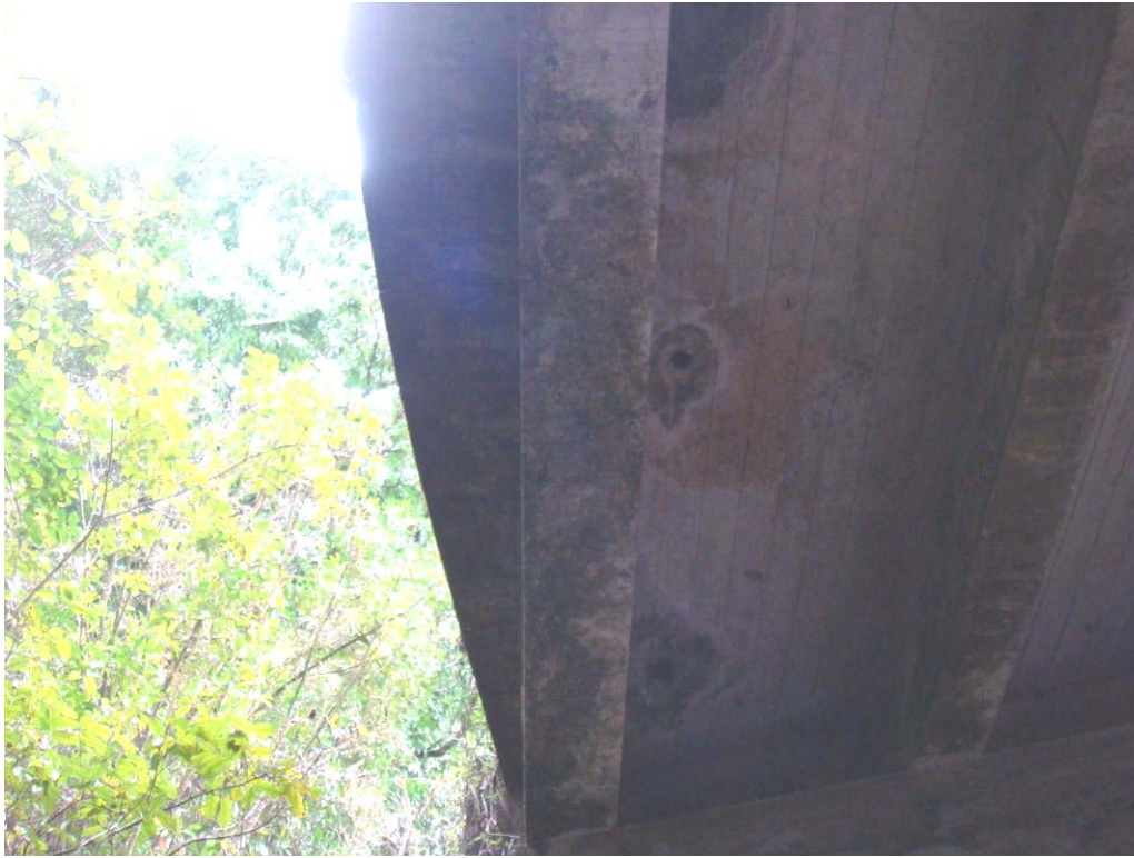
PHOTO 17 HAIRLINE LONGITUDINAL CRACK ALONG BOTTOM OF GIRDER G1
