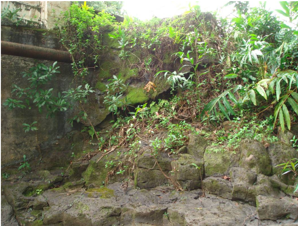
PHOTO 24 UNDERMINING AT UPSTREAM HANA CRM WALL
