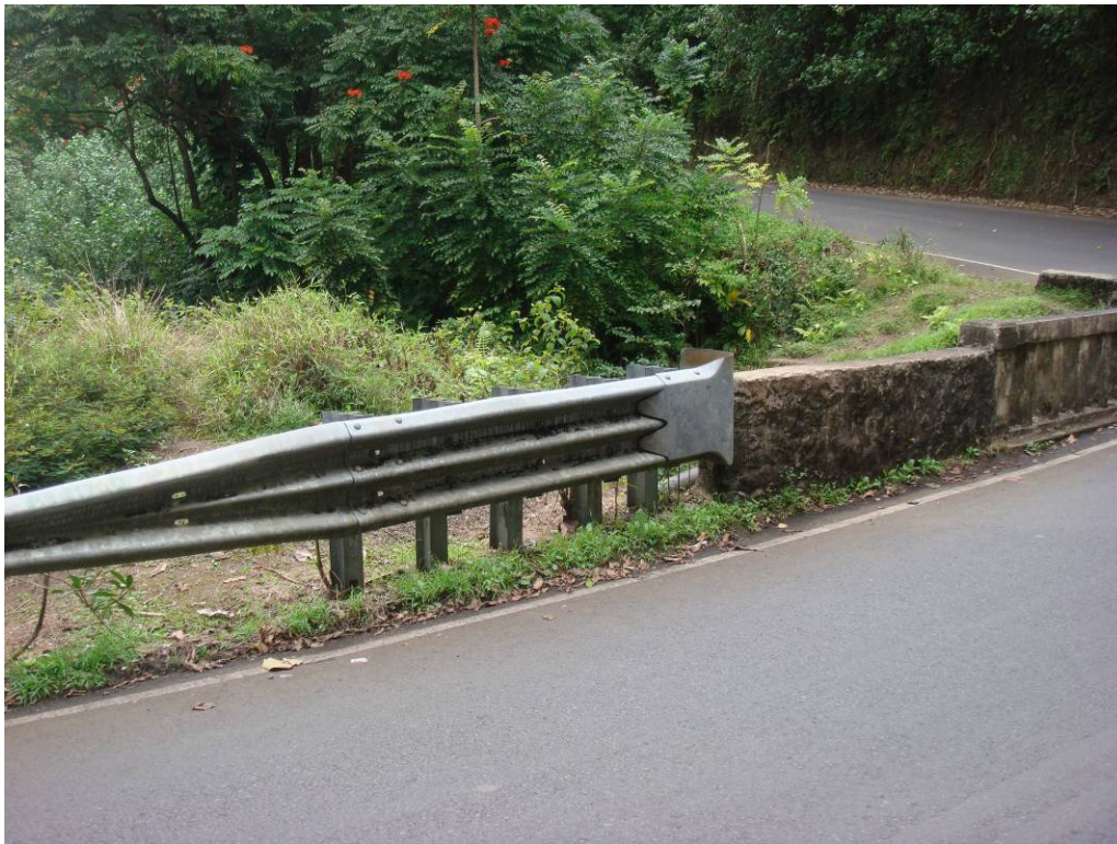
PHOTO 4 DOWNSTREAM / KAHULUI GUARDRAIL END TREATMENT AND CRM WALL. NOTE: GUARDRAIL END TREATMENT HT = 36"
