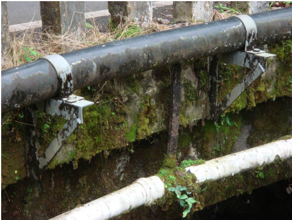
PHOTO 14 SUPPORTS FOR PVC PIPELINE ARE CORRODED ON THE DOWNSTREAM SIDE OF BRIDGE (SEE PHOTO 13)
