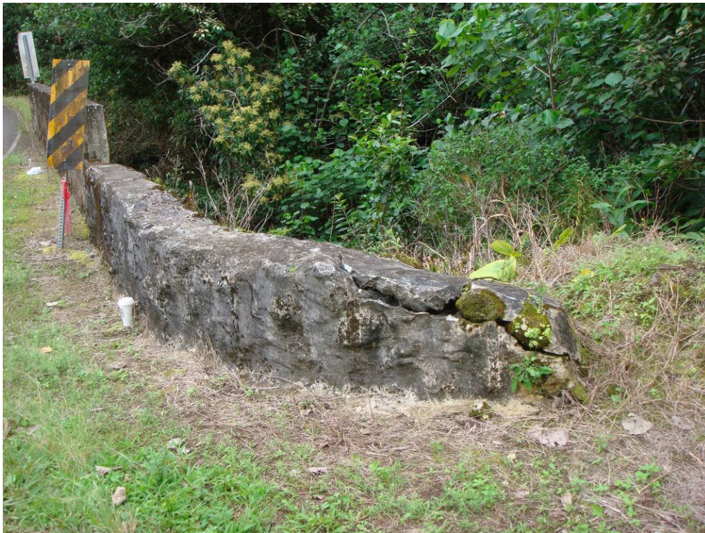
PHOTO 3 UPSTREAM / KAHULUI CRM WALL WITH COLLISION DAMAGE
