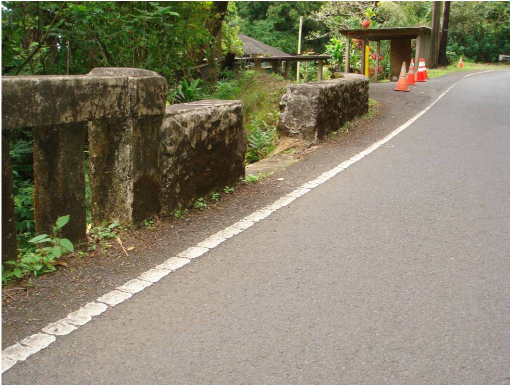
PHOTO 7 OPENING IN DOWNSTREAM HANA CRM WALL
