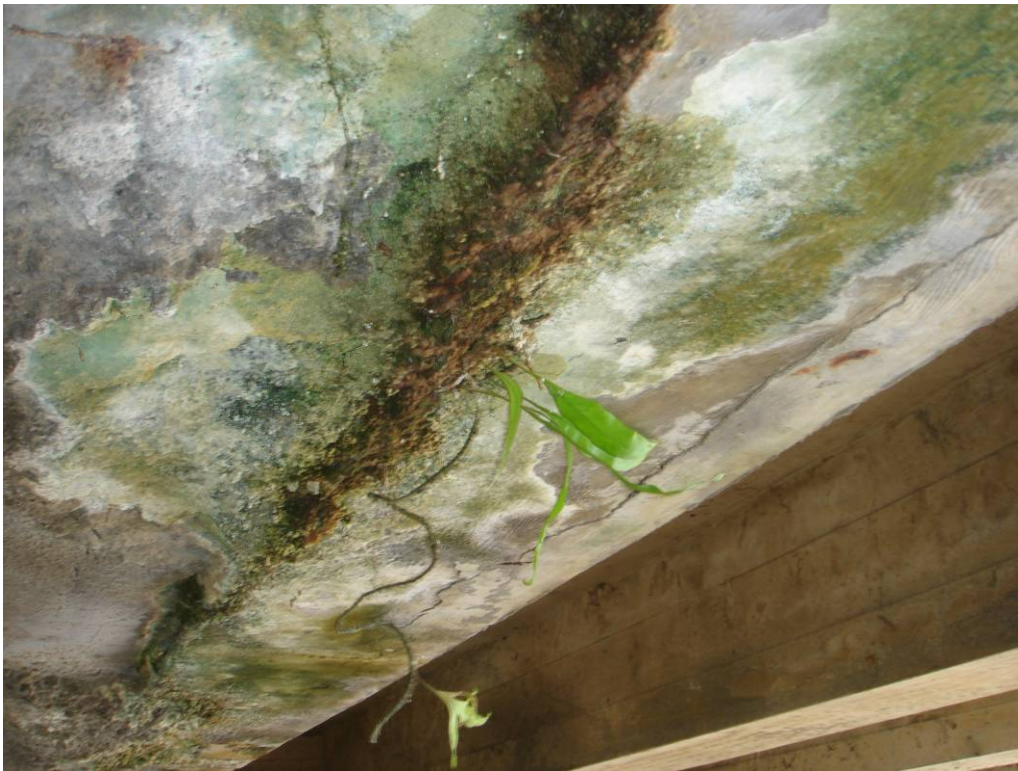
PHOTO 20 DELAMINATION AND VEGETATION GROWING IN GIRDERS G4 AND G5
