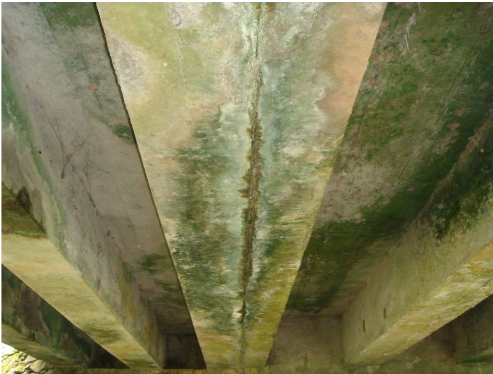
PHOTO 14 JOINT LEAKAGE IN SOFFIT LOOKING TOWARD KAHULUI WITH EFFLORESCENCE AND MOSS
