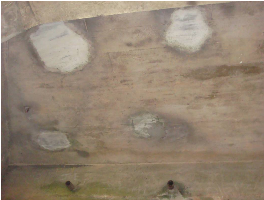
PHOTO 24 PATCHES IN SOFFIT NEAR HANA END
