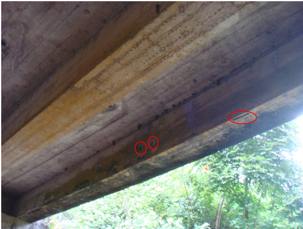
PHOTO 16 OVERALL VIEW OF GIRDER G8 LOOKING DOWNSTREAM WITH SEVERAL SMALL SPALLS WITH EXPOSED REBAR AND DELAMINATION THROUGHOUT THE UPSTREAM FACE
