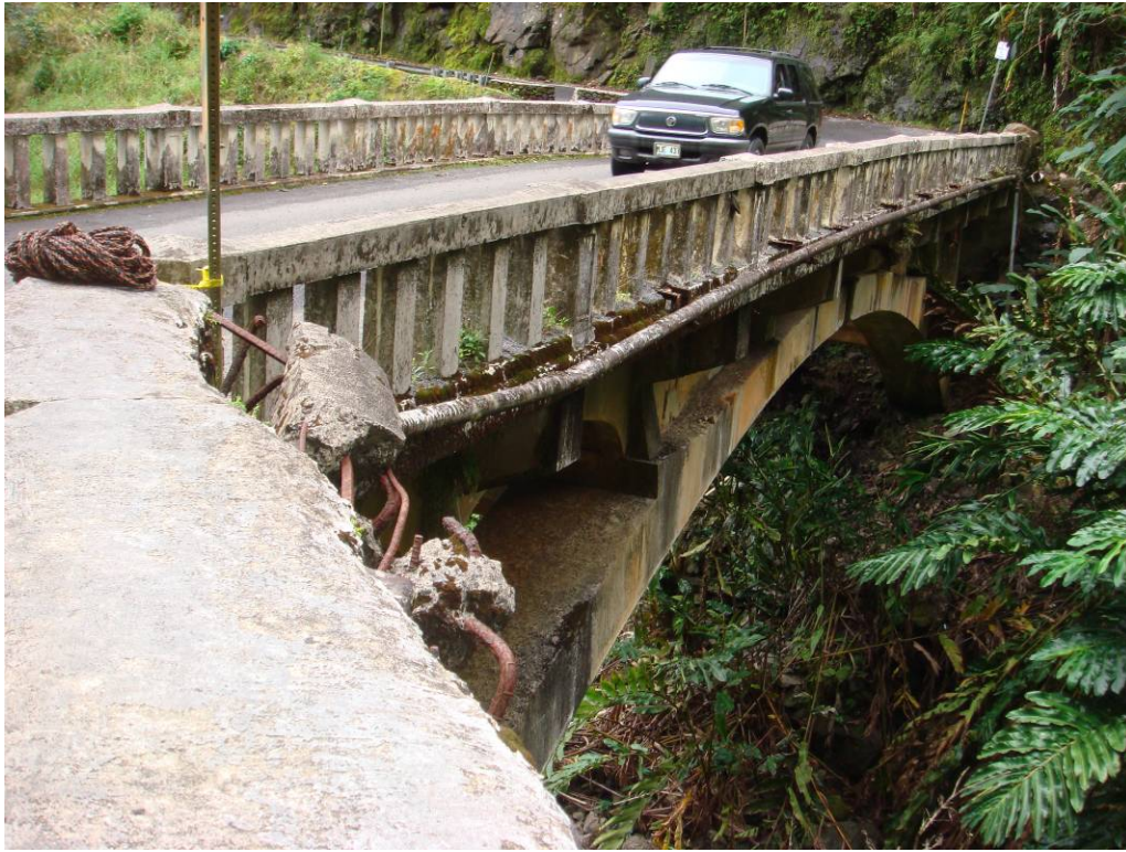
PHOTO 17 UPSTREAM ELEVATION AND UTILITY LINE ALONG BASE OF RAILING
