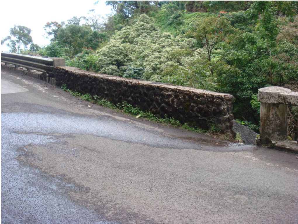
PHOTO 5 DOWNSTREAM / KAHULUI GUARDRAIL TRANSITION AND CRM WALL. NOTE: GUARDRAIL TRANSITION HT = 34"
