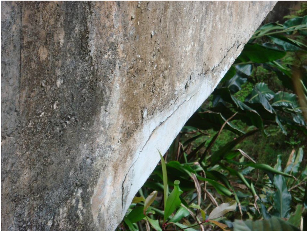
PHOTO 19 DELAMINATION (1' (H) X 3' (W)) IN DOWNSTREAM FACE OF ARCH RIB UNDER DOWNSTREAM / HANA SPANDREL COLUMN
