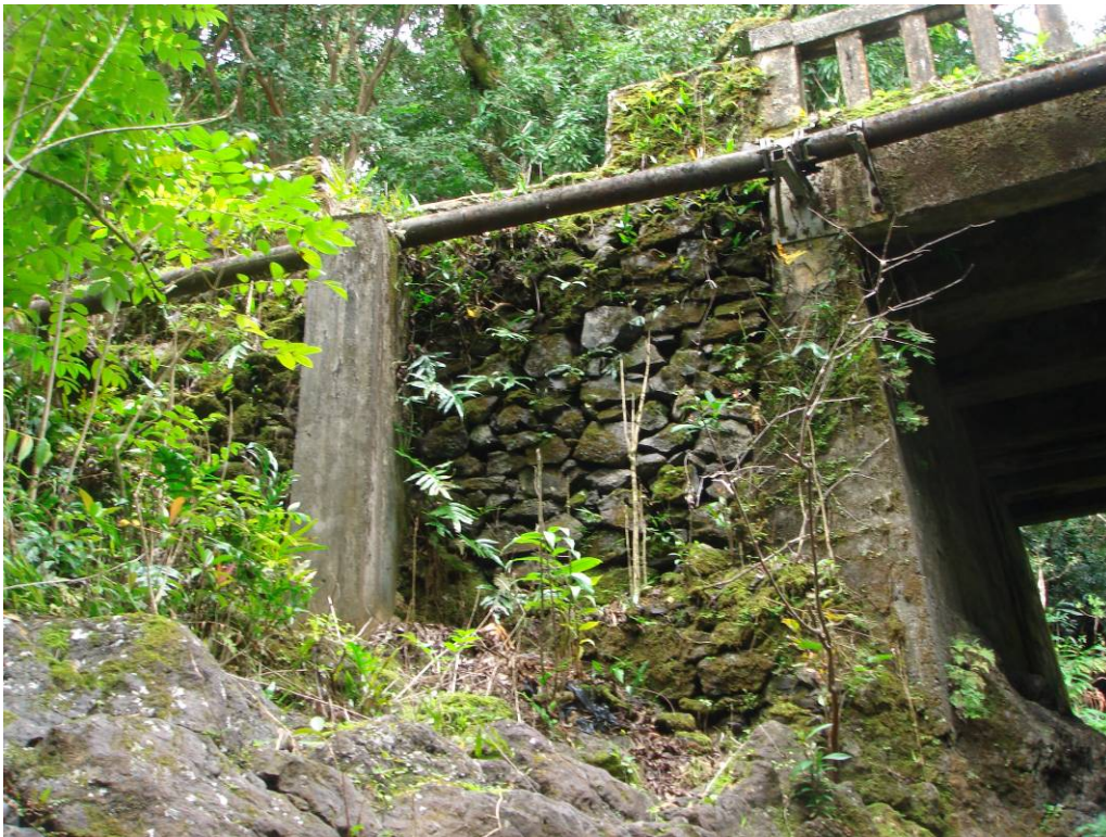
PHOTO 20 DOWNSTREAM HANA CRM WINGWALL AND UTILITY PIPE
