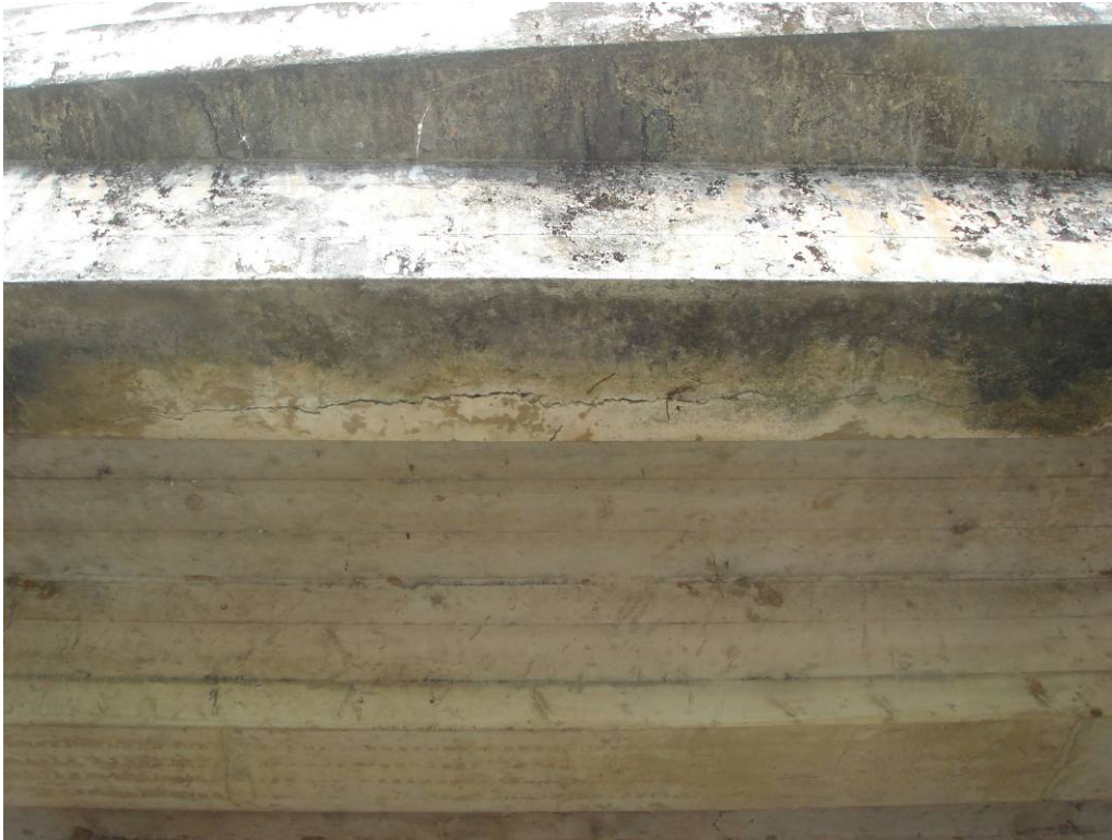
PHOTO 17 6' DELAMINATION IN GIRDER G8
