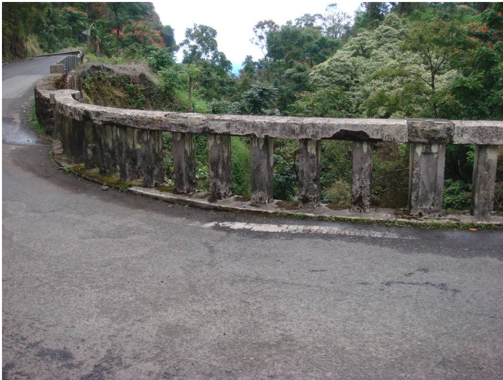
PHOTO 10 PARTIAL VIEW OF DOWNSTREAM RAILING ELEVATION NEAR KAHULUI. NOTE: RAILING HT = 33"
