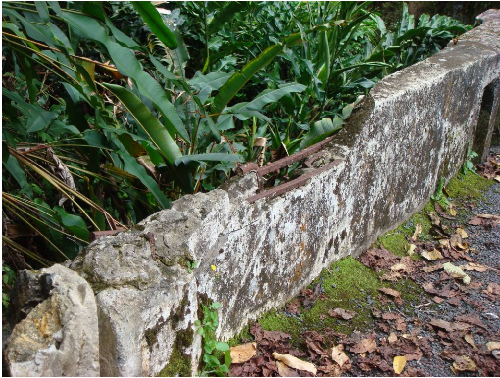
PHOTO 7 CLOSE UP OF COLLISION DAMAGE AT UPSTREAM / HANA CONCRETE PARAPET
