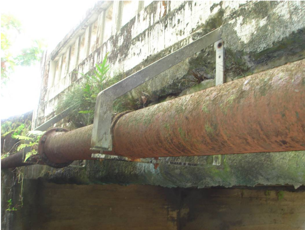
PHOTO 11 CLOSE UP OF UTILITY PIPE AND HANGERS ON UPSTREAM SIDE OF BRIDGE
