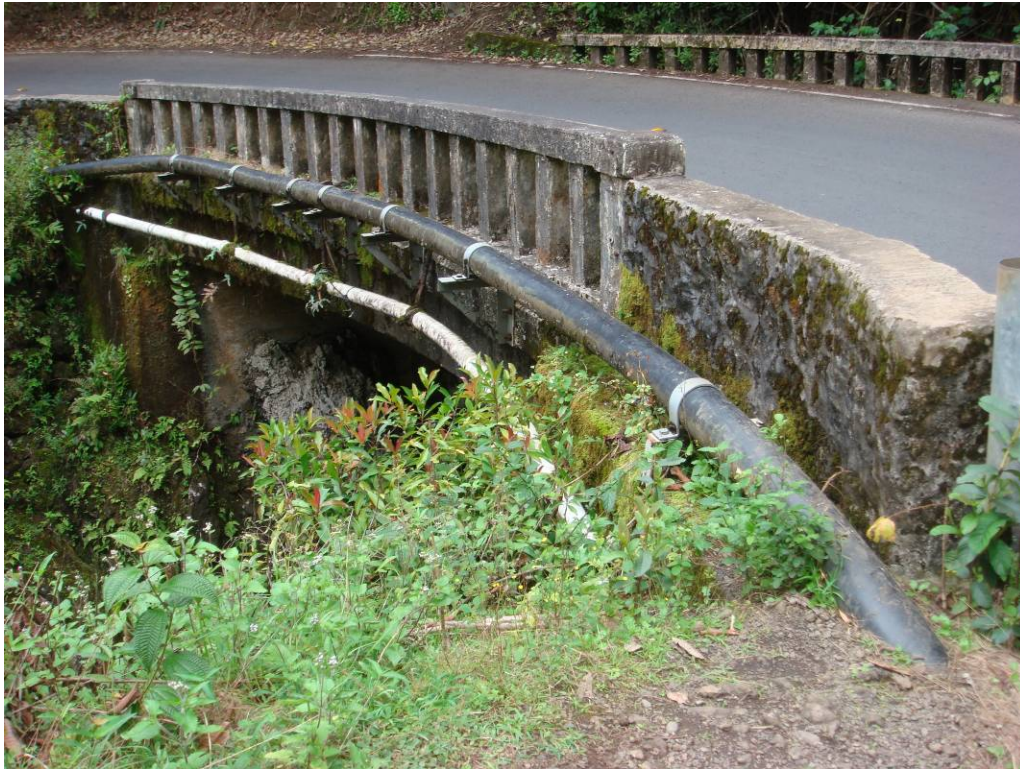
PHOTO 13 DOWNSTREAM BRIDGE ELEVATION, BACKSIDE OF DOWNSTREAM BRIDGE RAILING AND CRM WALLS, AND UTILITY LINES ATTACHED TO SIDE OF BRIDGE
