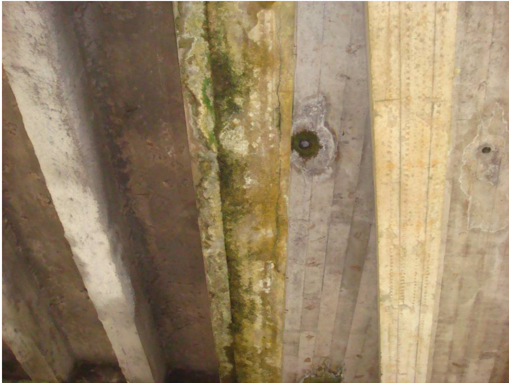
PHOTO 15 DELAMINATION AND HAIRLINE CRACK (8' LONG) IN BOTTOM OF GIRDER G5 NEAR HANA ABUTMENT
