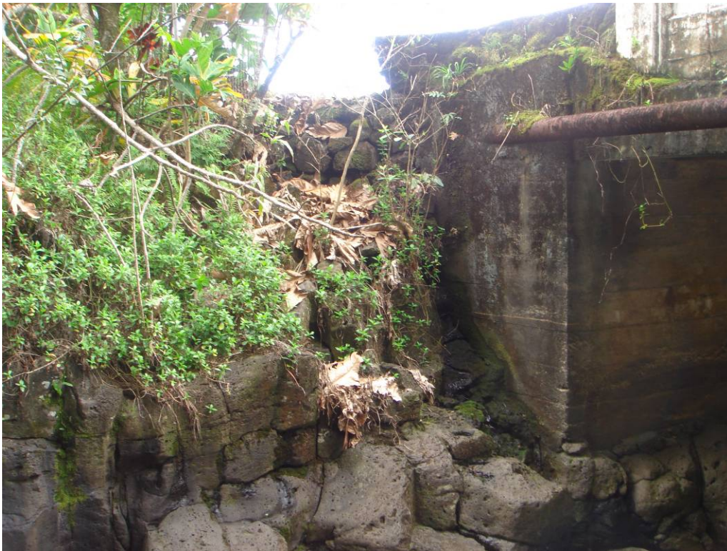
PHOTO 26 LOOSE ROCKS IN UPSTREAM KAHULUI CRM WALL
