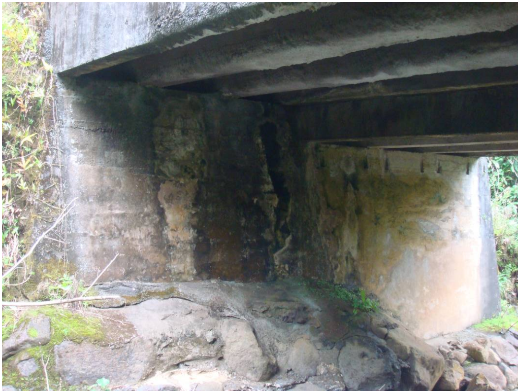
PHOTO 18 KAHULUI ABUTMENT WITH DARK WATER STAINS
