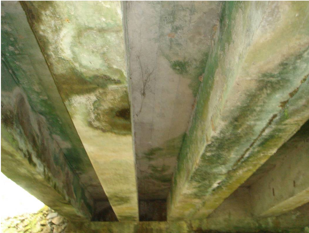
PHOTO 13 UPSTREAM HALF OF SOFFIT LOOKING TOWARD KAHULUI WITH EFFLORESCENCE AND MOSS. DELAMINATION IN GIRDER G4 NEAR HANA ABUTMENT AND VERTICAL CRACKS.
