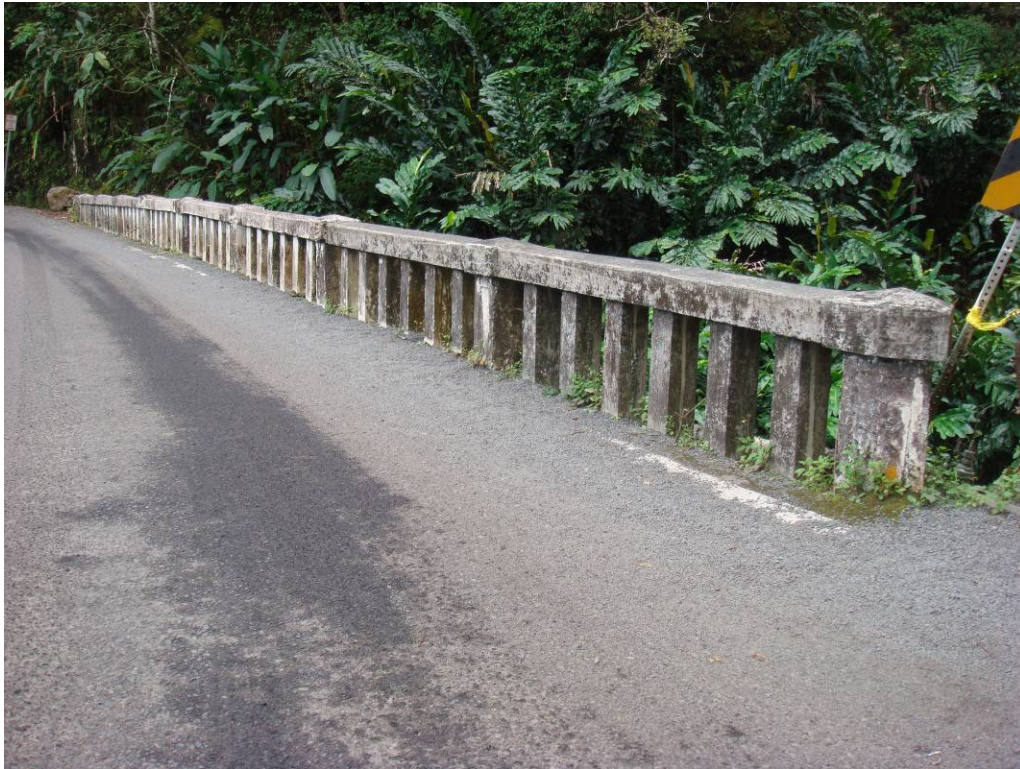
PHOTO 9 UPSTREAM RAILING ELEVATION. NOTE: RAILING HT = 29"
