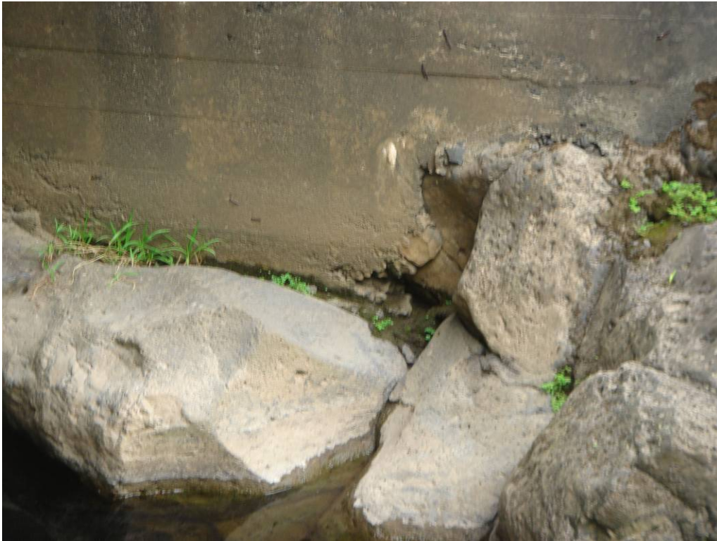
PHOTO 29 MINOR UNDERMINING AT DOWNSTREAM END OF KAHULUI ABUTMENT
