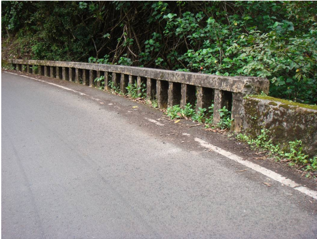
PHOTO 7 UPSTREAM BRIDGE RAILING. NOTE: RAILING HT = 24"
