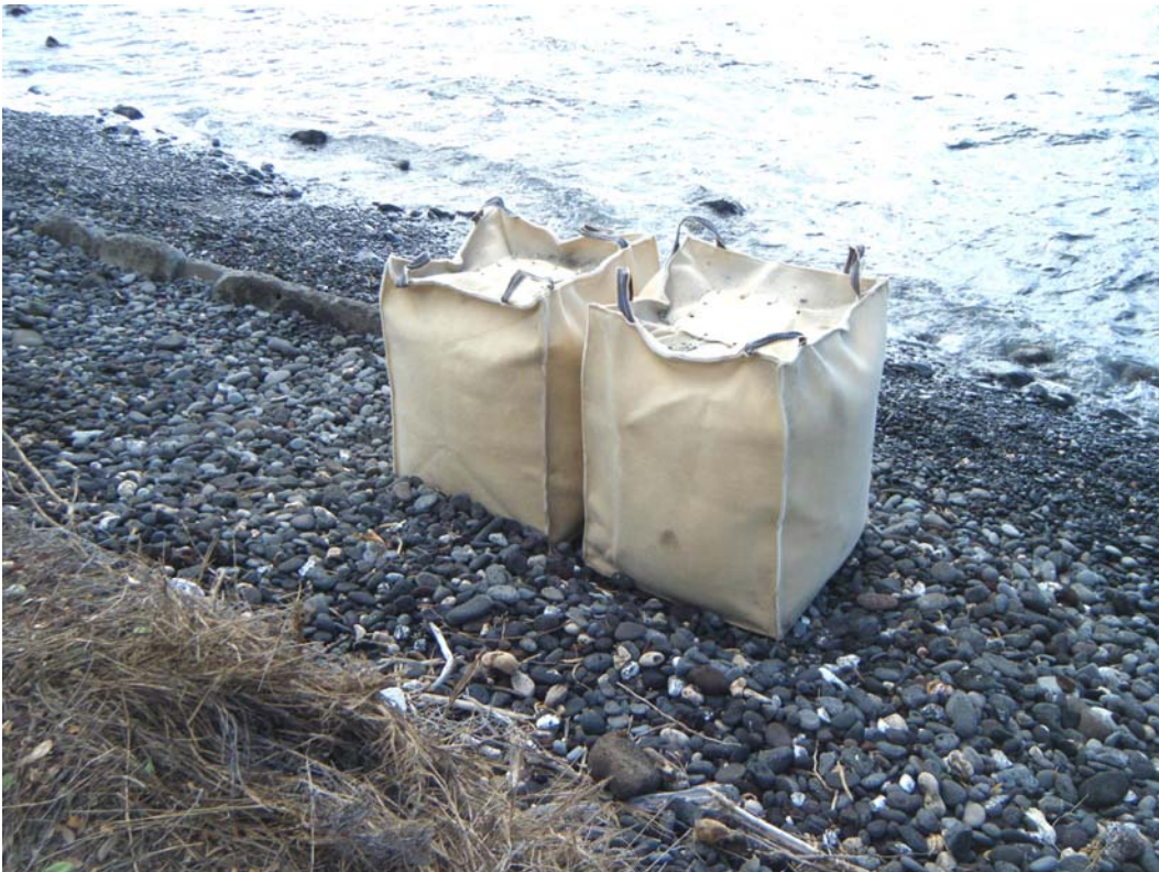
Gravel bags to be lined up to form barrier
