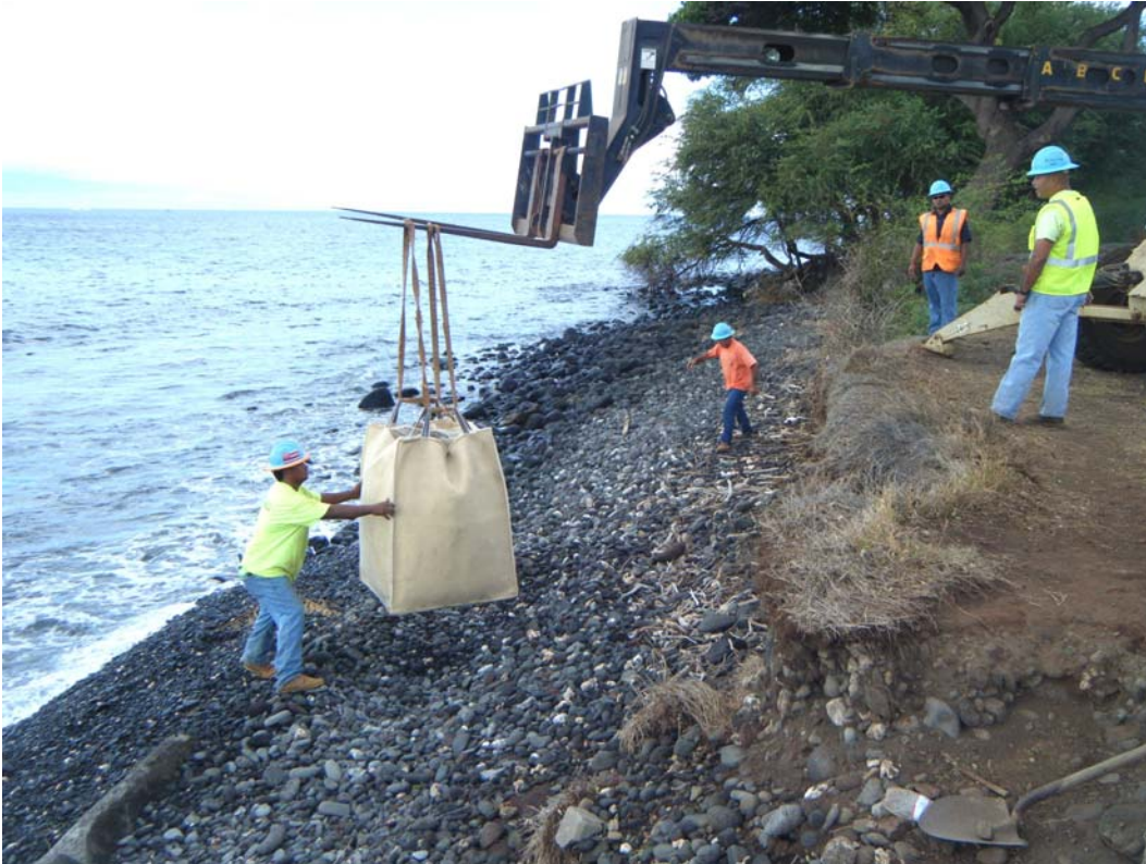
Filled gravel bags mechanically lowered into place
