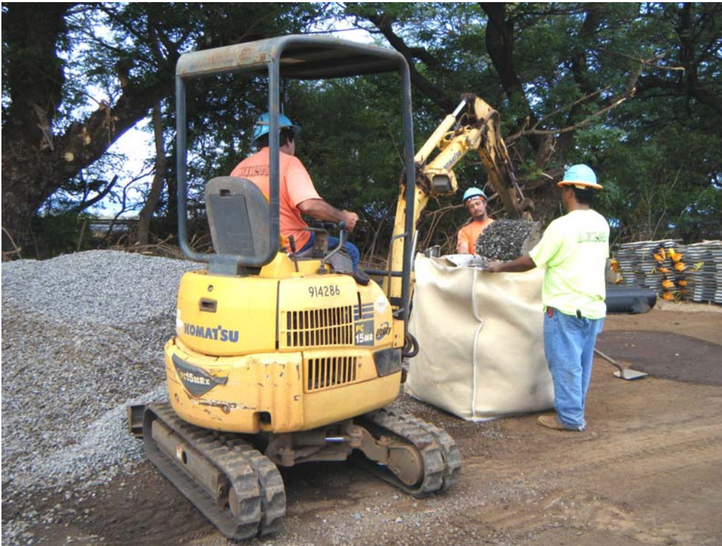
High strength geotextile bags filled with clean gravel off-site
