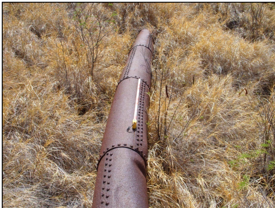
Figure 44. Picture showing a section of 24-inch riveted pipe located atop Site -5950 Feature 26.
