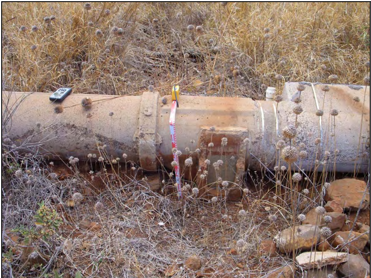
Figure 46. Picture showing a section of the 16-inch concrete pipe (CSH 5).
