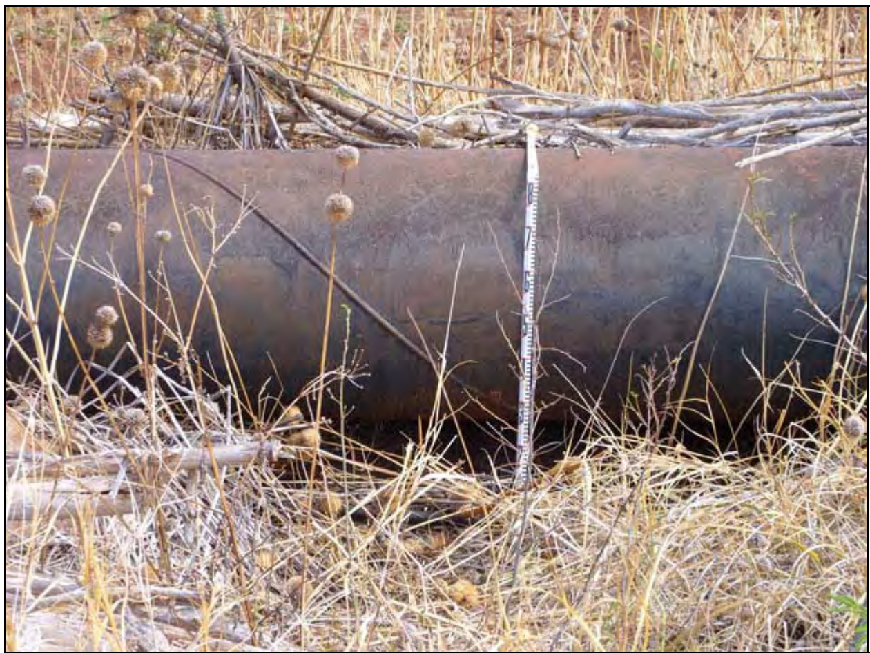
Figure 42. Picture showing the 24-inch creosote covered irrigation pipe (CSH 4).
