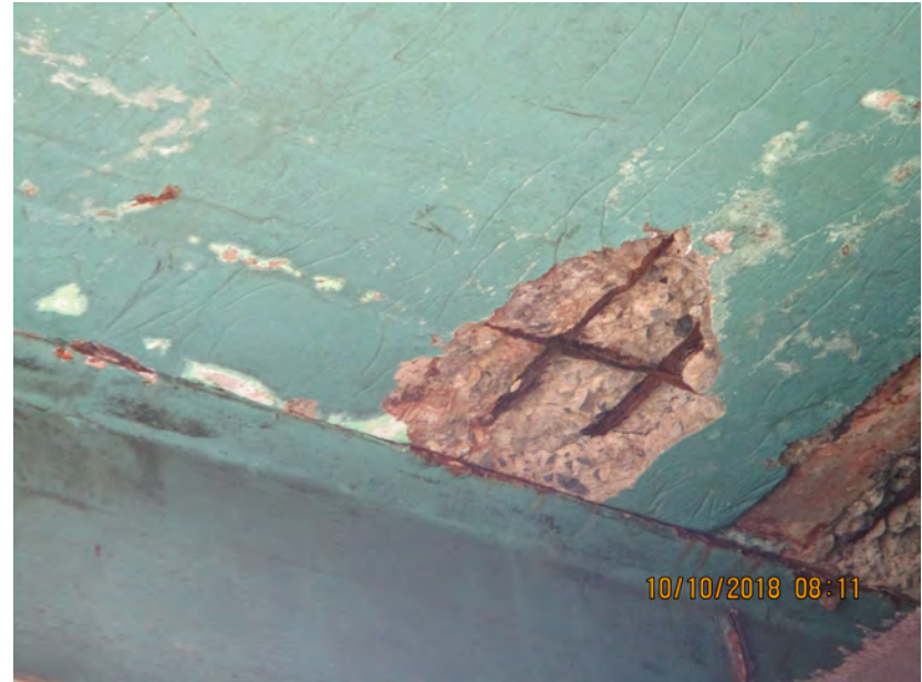
Photo 6: View of light green paint on concrete underneath damaged Ele'e Shopping Center pedestrian bridge.
