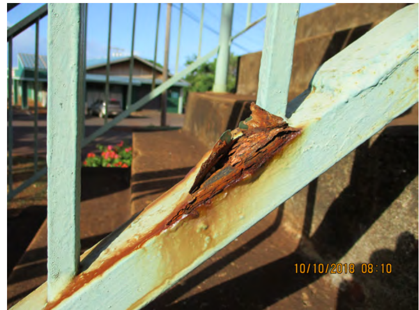
Photo 4: Close-up view of damaged section on metal hand railing.
