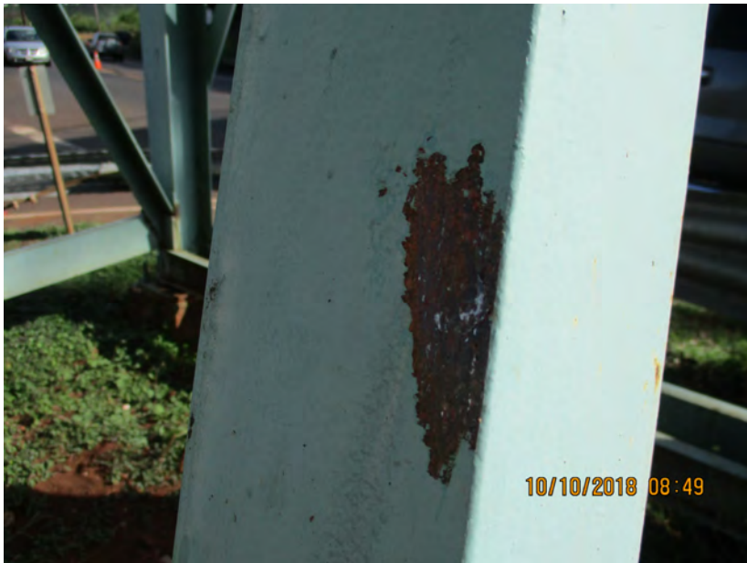
Photo 7: View of paint sample location on steel bridge support showing light green paint over red primer.
