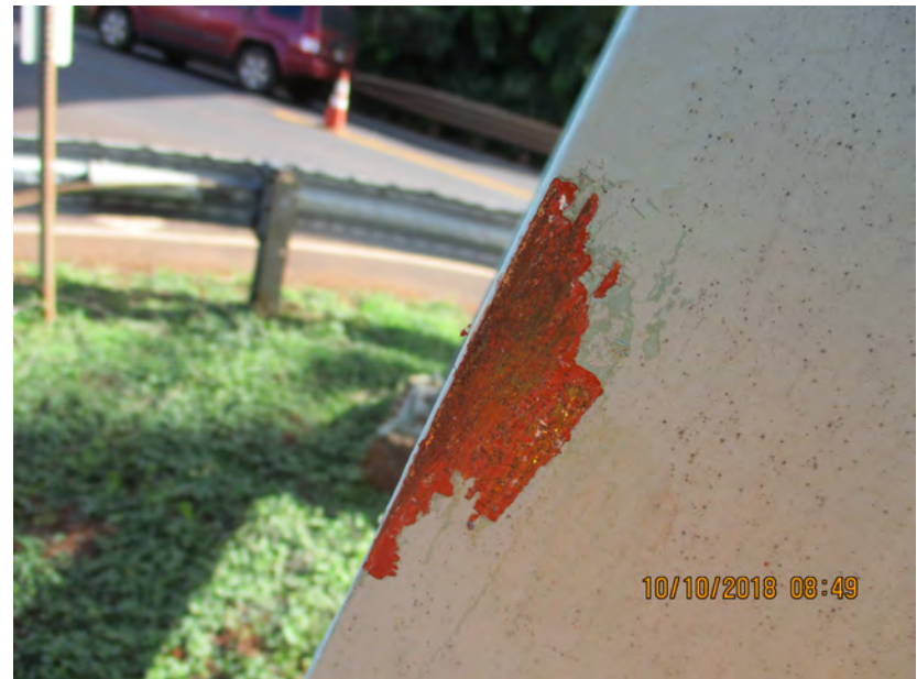
Photo 8: View of paint sample location on steel bridge support showing light green paint over red primer.
