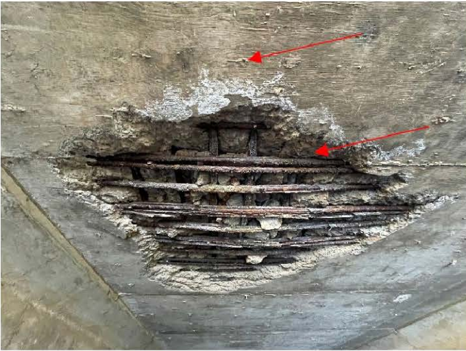
60 S.F. Spall in Soffit (Polihale Cell) *Overhead
