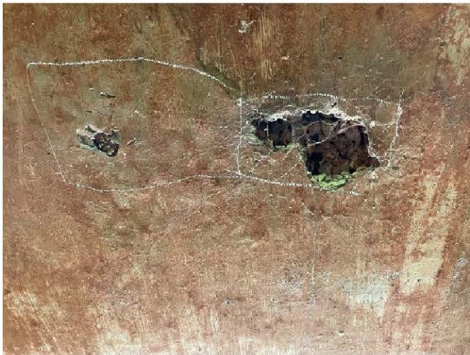
2 S.F. Spall in Soffit (Cell #4), Type 1 Repair *Overhead
