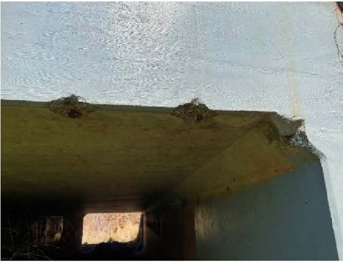
(3) Spalls in Bottom Edge of Headwall (Cell #1), Type 3 Spall Repair (a=12", b=6", length=12", each) *Overhead
