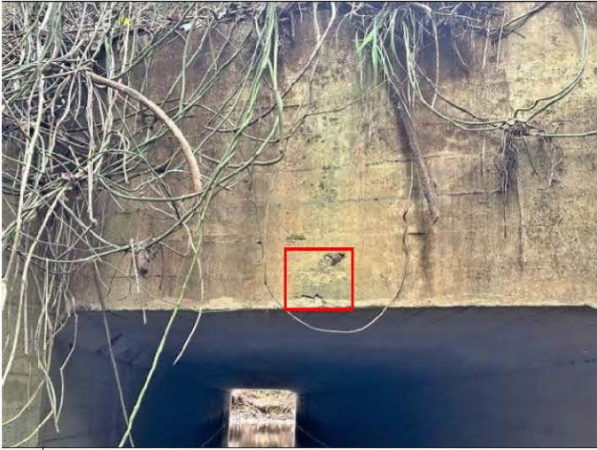
3 S.F. Spall in Bottom of Upstream Headwall, Type 1 Repair *Overhead
