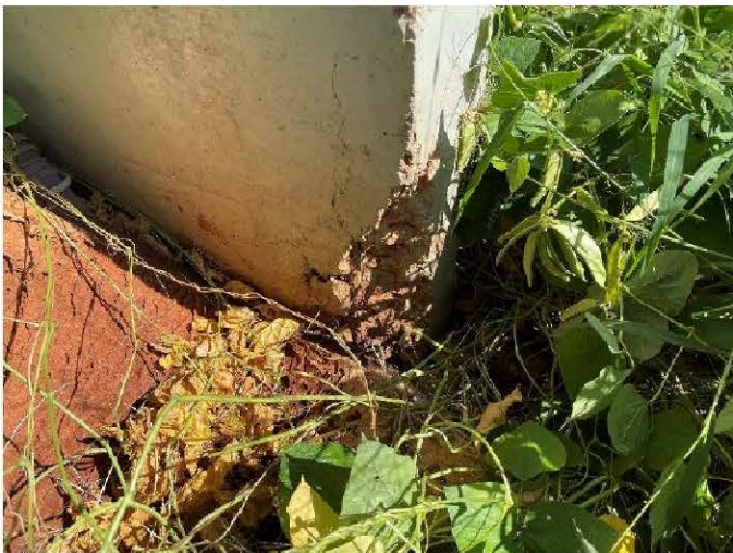
2 L.F. Spall in Leading Edge of Wall (Cell #4), Type 2 Repair (a=12", b=9") *At your feet
