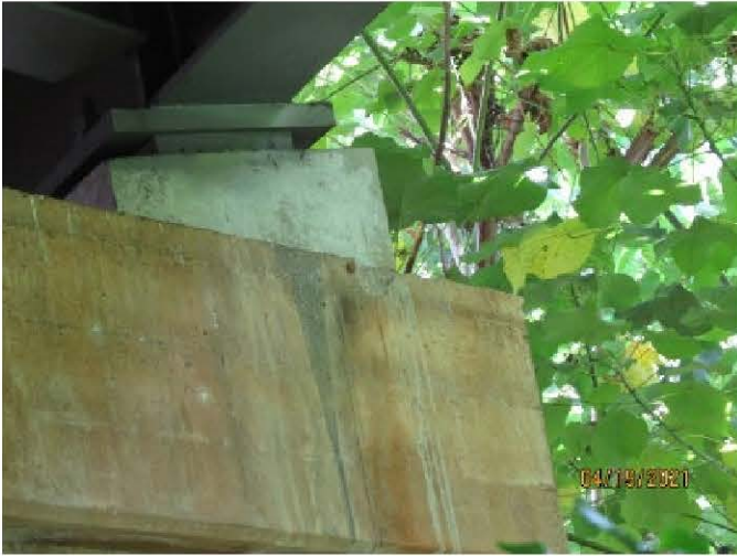
1'-0" Long Spall in Top edge of Pilecap. Type 3 Spall Repair (a=9", b=9"). *Overhead
