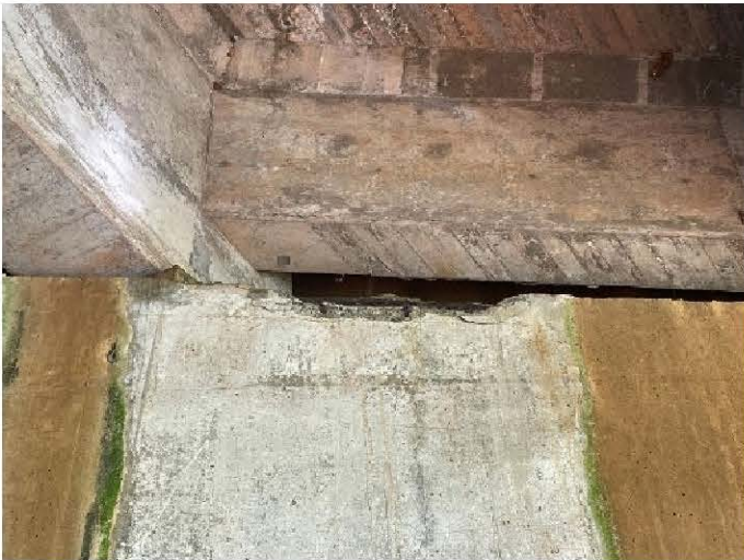
4 S.F. Spall at Top of Abutment Wall Between Girders 2 and 3, Type 3 Repair *Overhead
