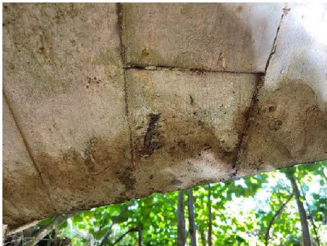
2 S.F. Spall in Soffit of Downstream Headwall, Type 1 Repair *Overhead
