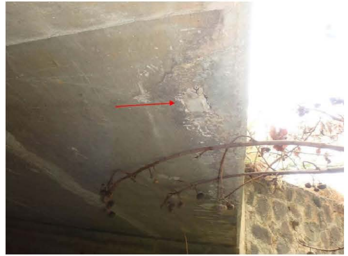
8 S.F. Spall in Headwall (Polihale Cell), Type 1 Repair *Overhead
