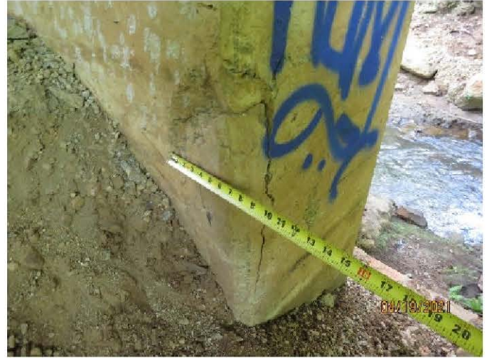
2'-0" Long Spall in Downstream Nose of Pier at Bottom. Type 3 Spall Repair (a=12", b=12"). *At your feet
