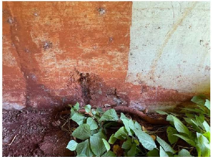
2 S.F. Spall at Bottom of Culvert Wall (Cell #4), Type 1 Repair *At your feet
