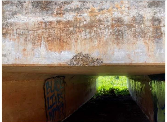
2 S.F. Spall at Bottom of Culvert Wall (Cell #4), Type 1 Repair *At your feet
