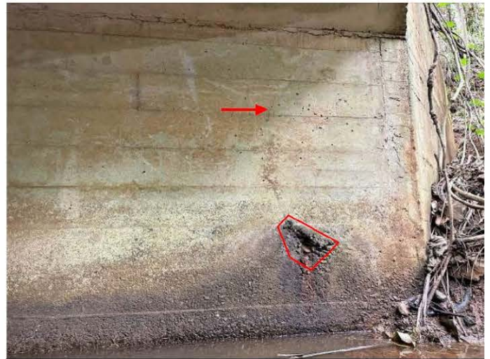
2 S.F. Spall in Bottom of Upstream Headwall, Type 1 Repair * Vertical
