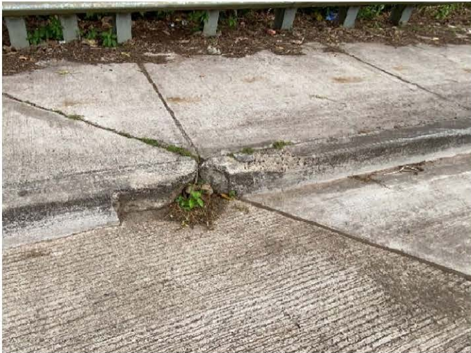
4'-0" Long Spall in Curb at Joint. Type 3 Spall Repair (a=9", b=6"). Provide Expansion Separation at Joint. *At your feet
