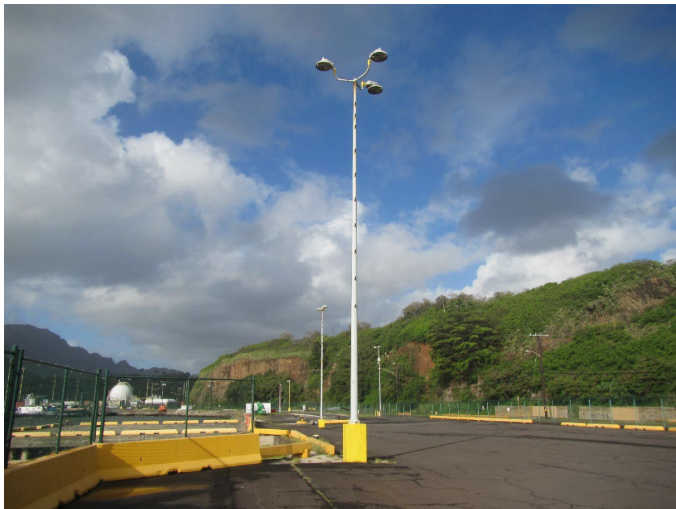
Photo 2: Typical Pier 2 Pole (Pole PP-1 Shown, Pole PP-2 Beyond)
