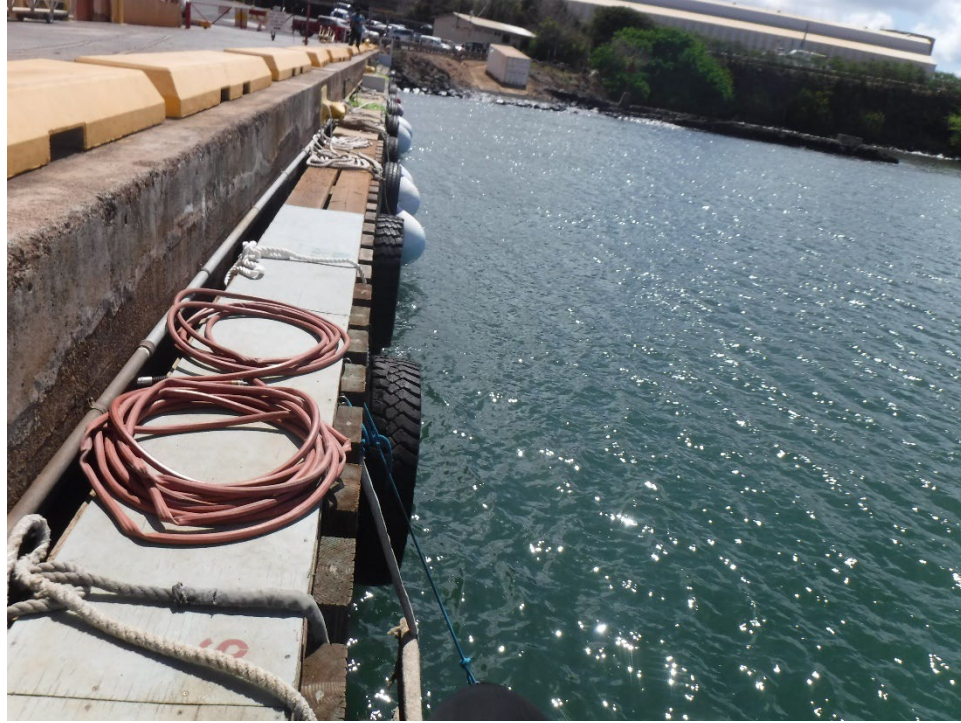
Photo 5: Fender System and Waterline
