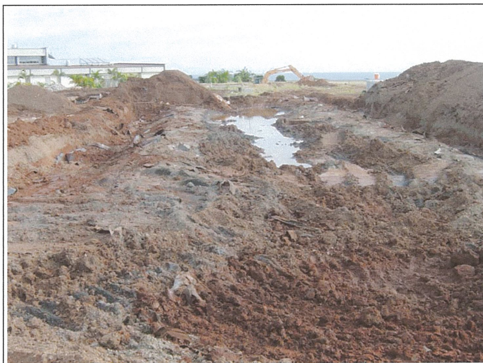
Photograph 3: Trenchline of UST piping to burn pit area.
