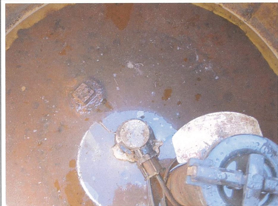
Photograph 2: Manhole accessway for fill pipe.
