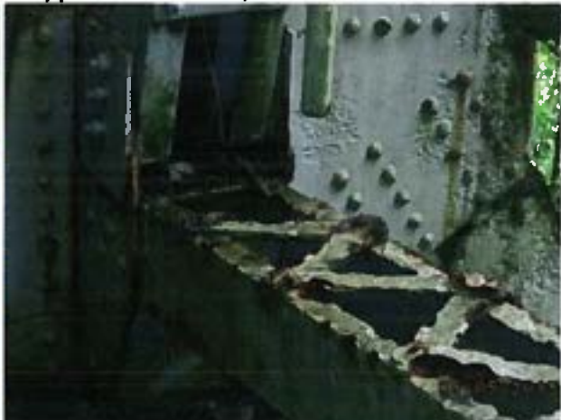
Bottom of bent 7 outlet end, column brace plates and lacings has corrossions.
