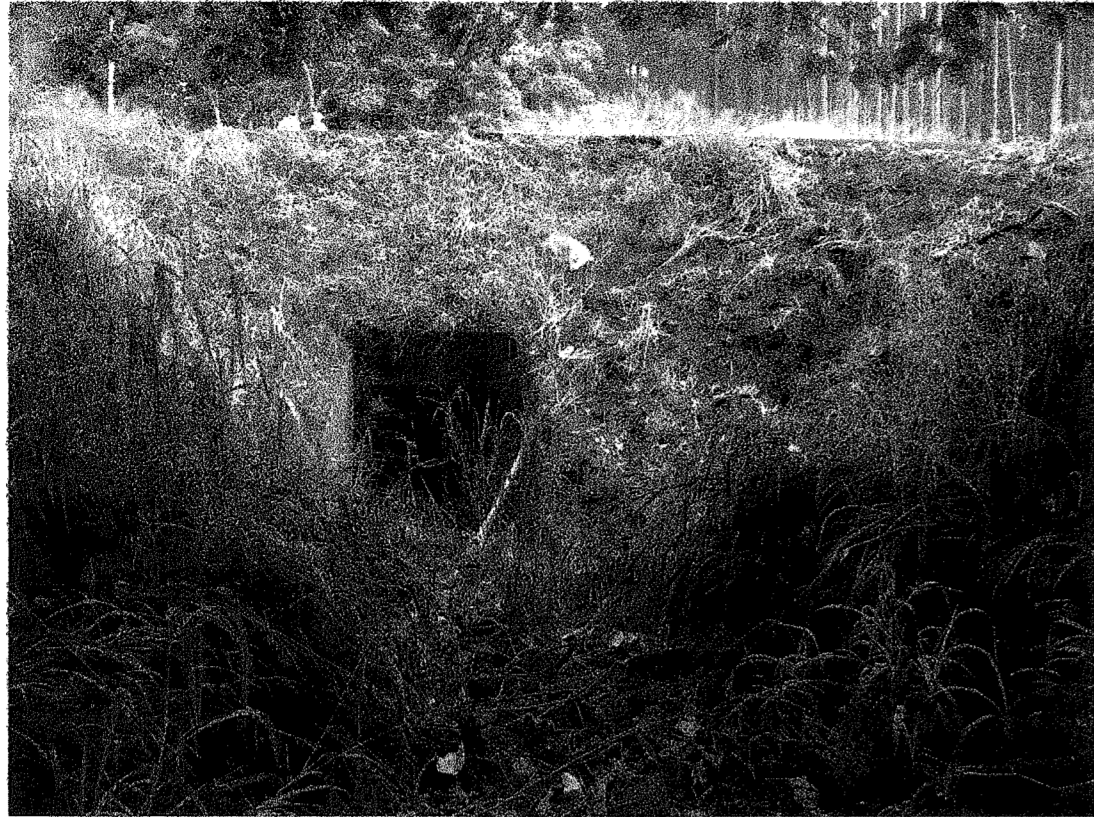
Photo 1 Remove silt deposit & loose vegetation
