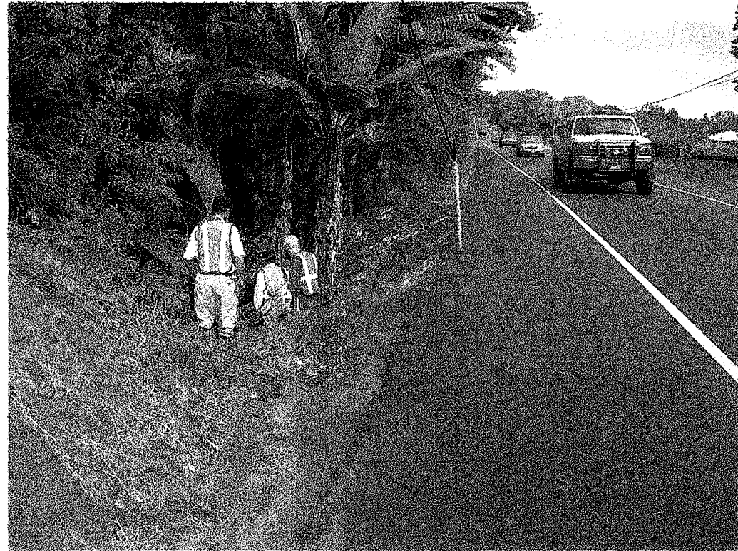
Photo 1 Clear loose debris from above & around inlet opening
