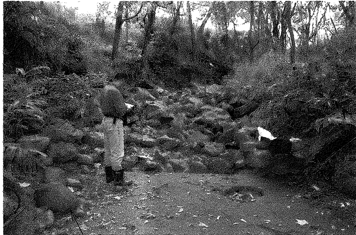
Photo 1 Remove loose rocks Repair slope embankment Remove loose rocks
