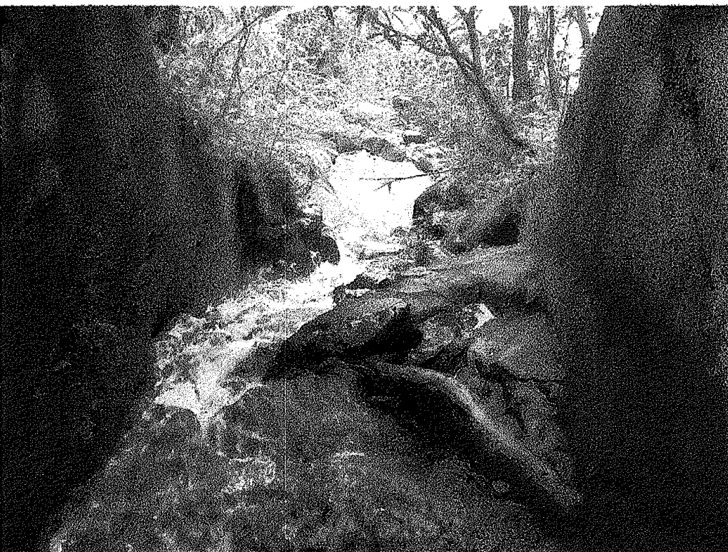
View looking downstream from within culvert
